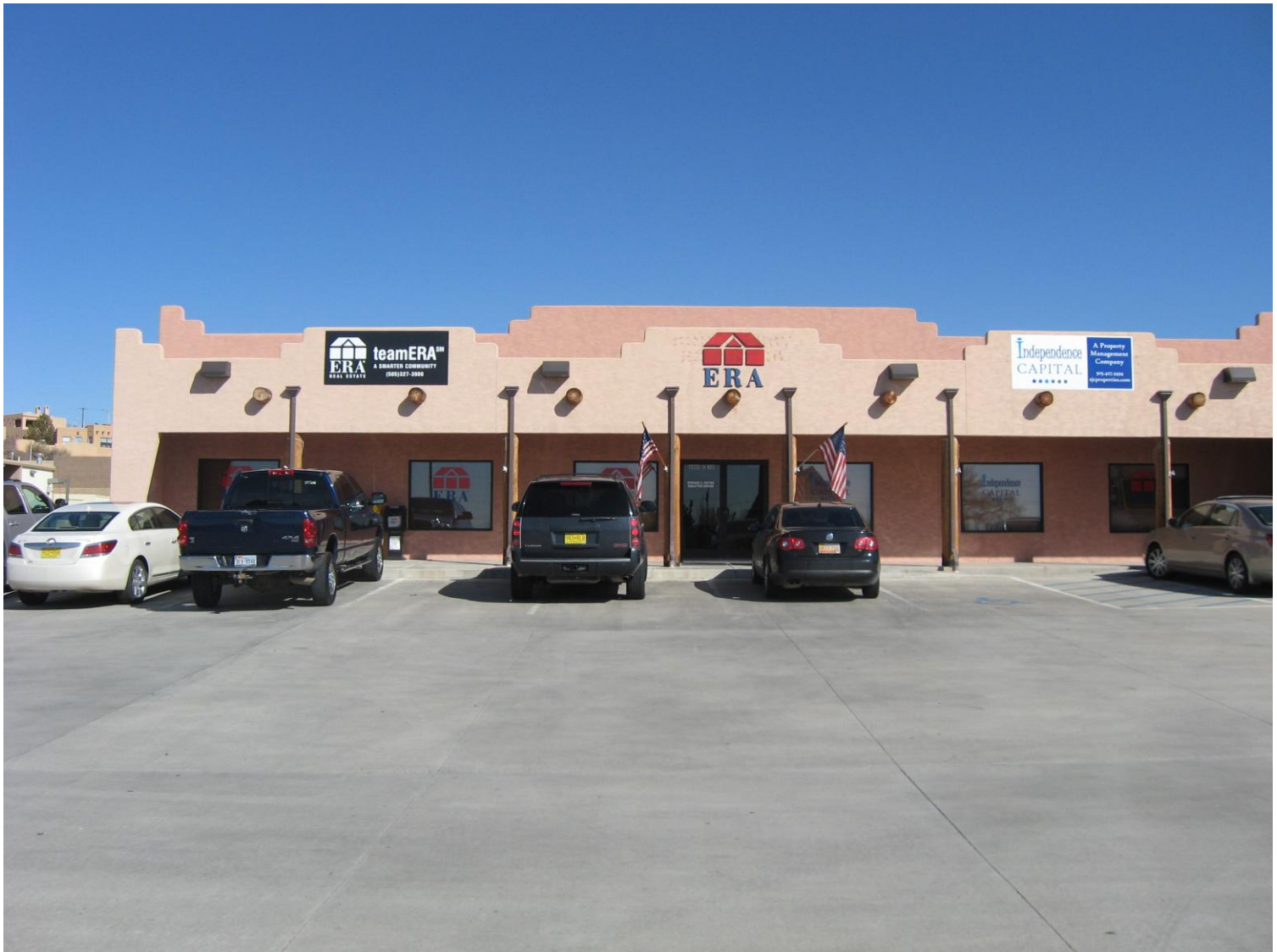
Front of structure looking North 2/28/13
