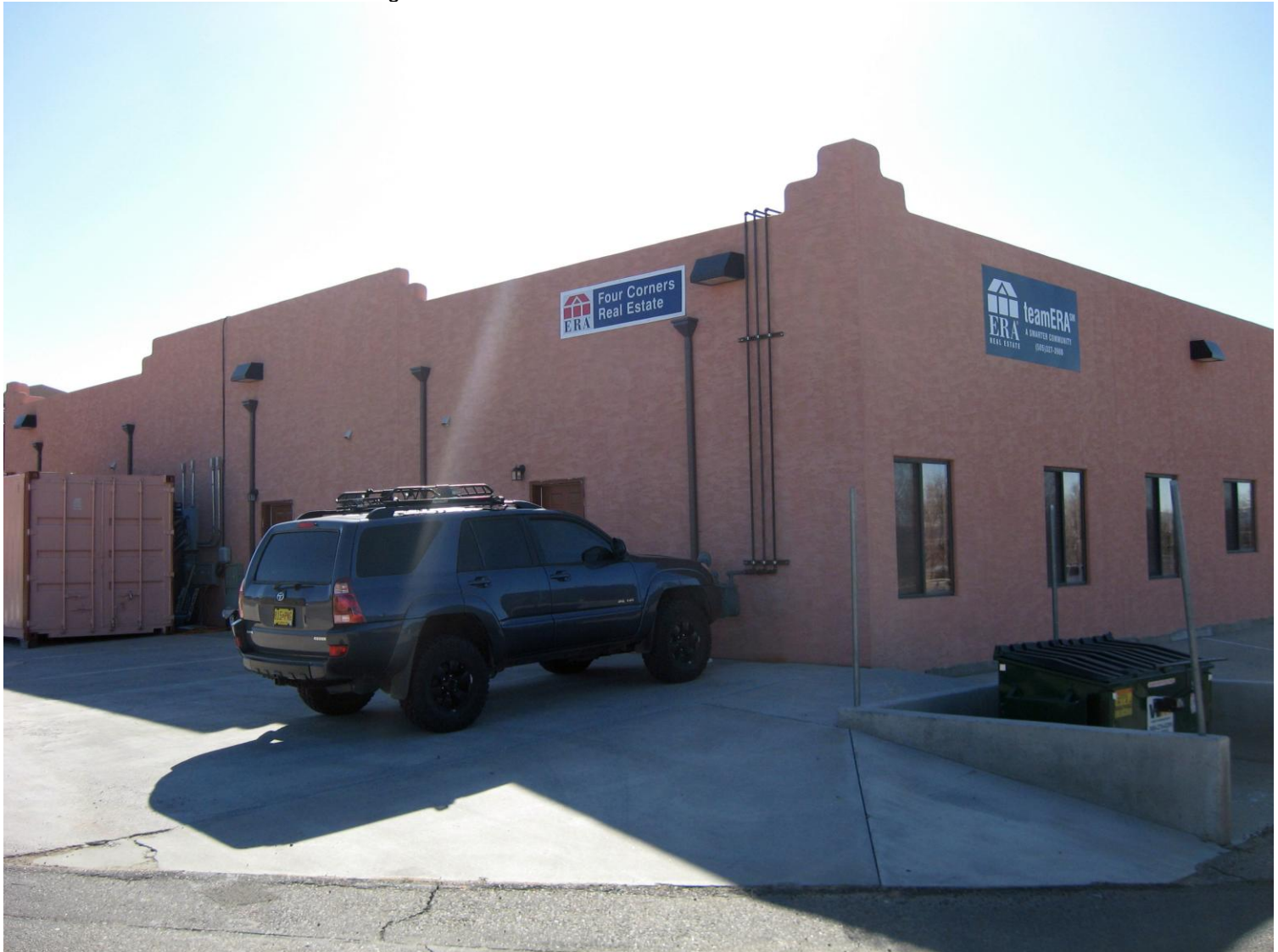
Back and West side of structure looking SE 2/28/13
