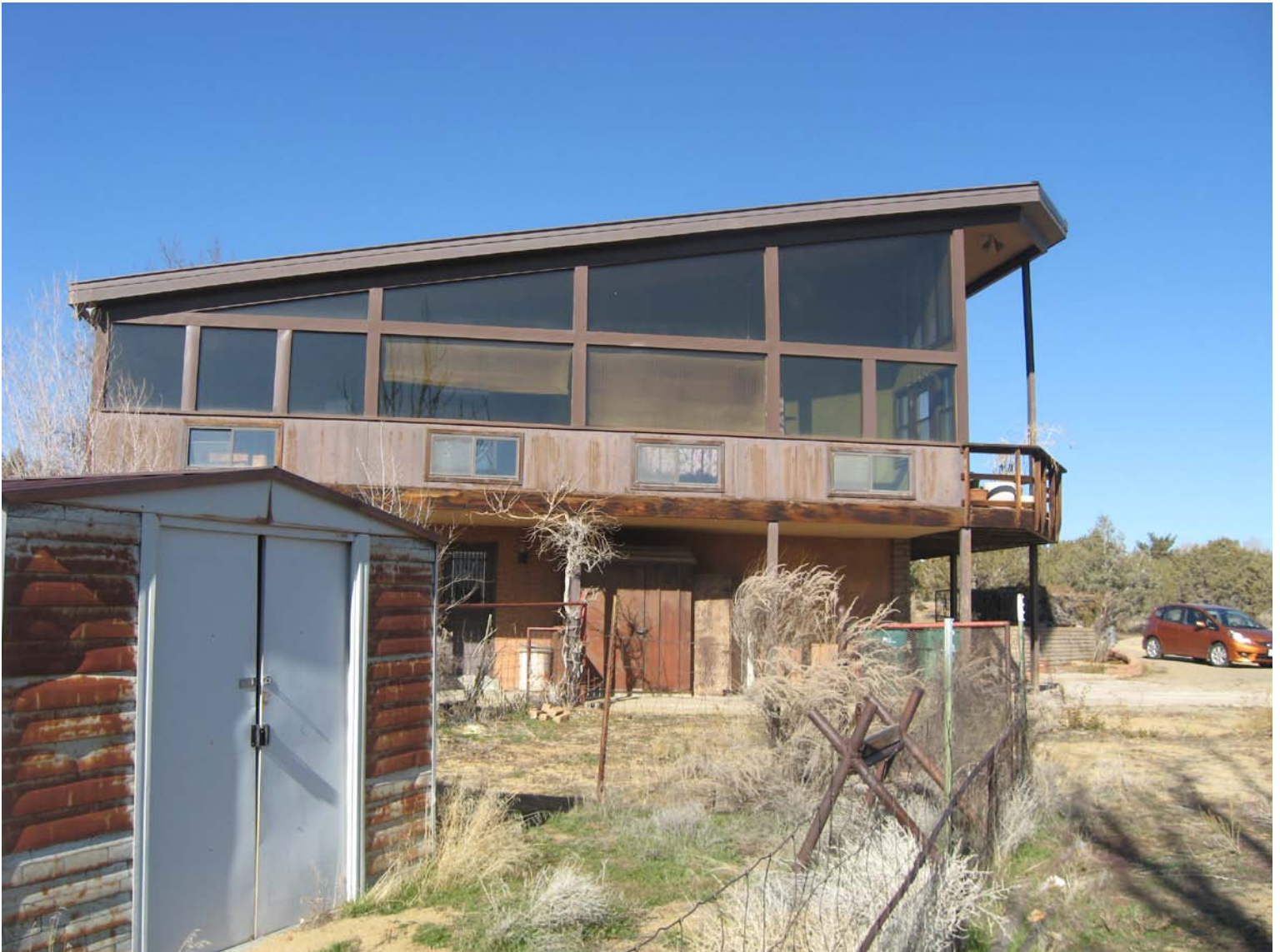
Side of structure looking North
