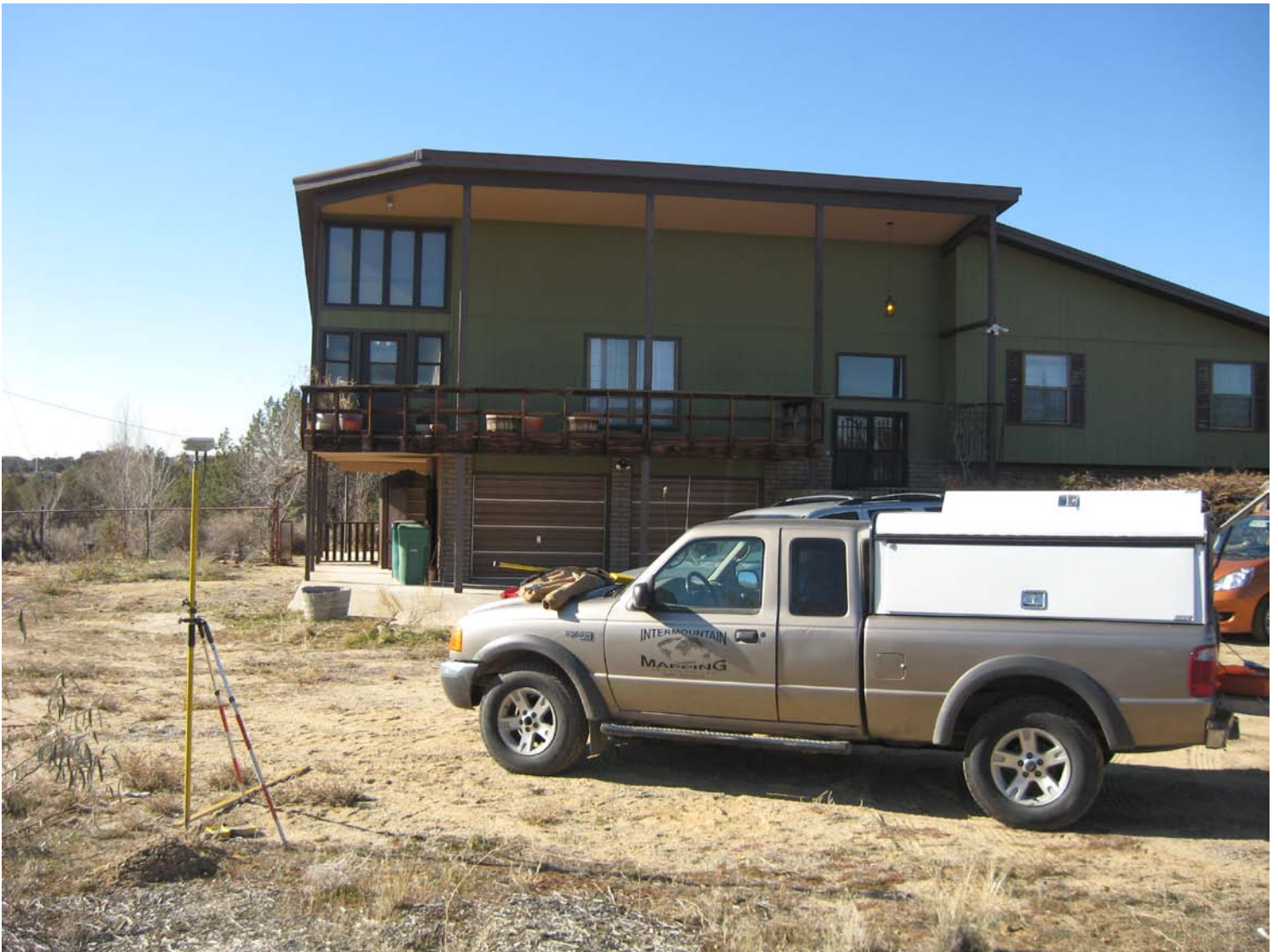
Front of structure, looking West.
