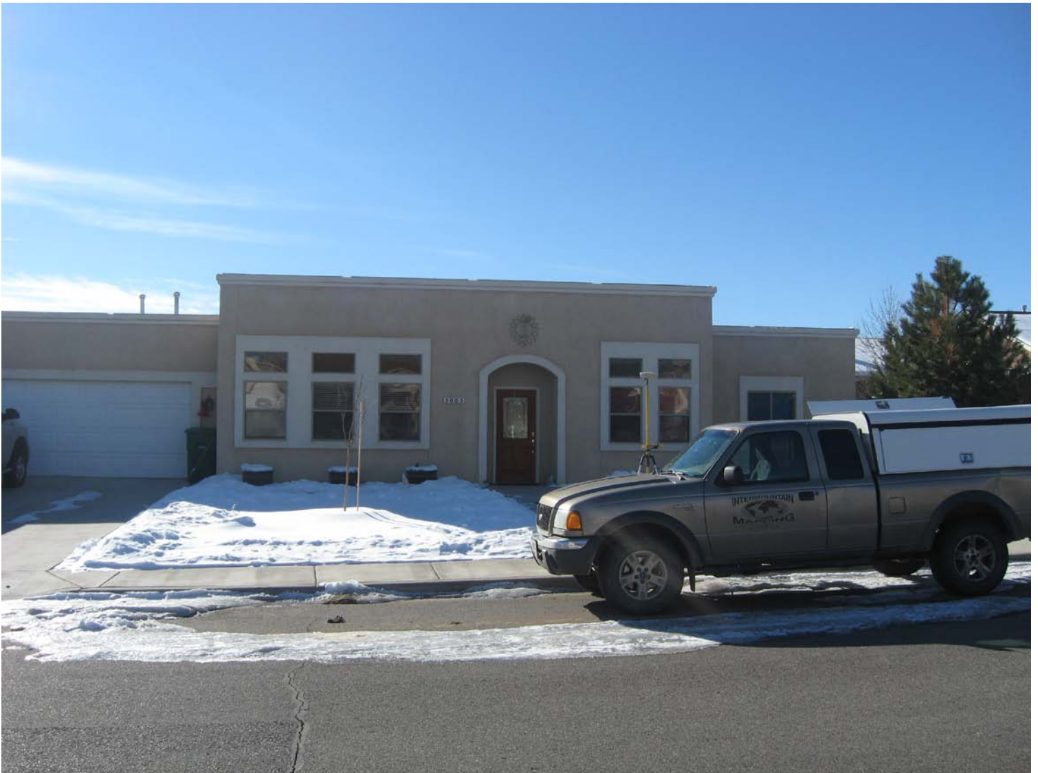
Front of House looking South
