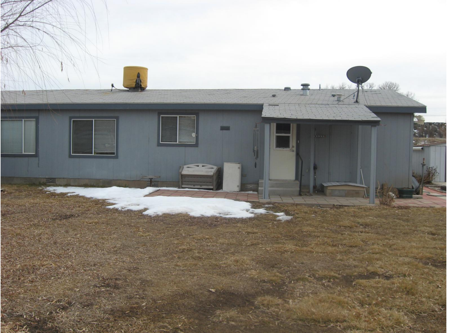
Back of structure looking East
