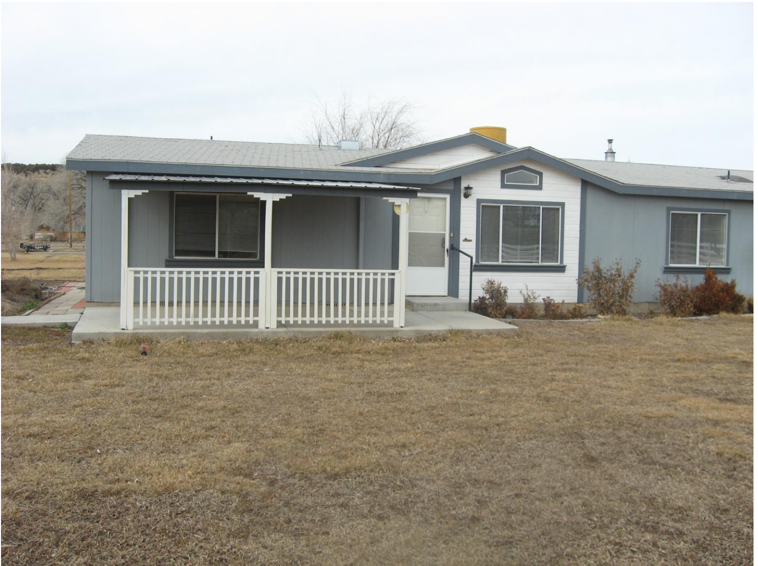
Front of structure looking West
