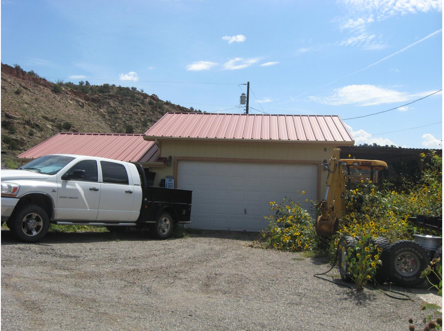
Front of structure looking South 9/9/13
