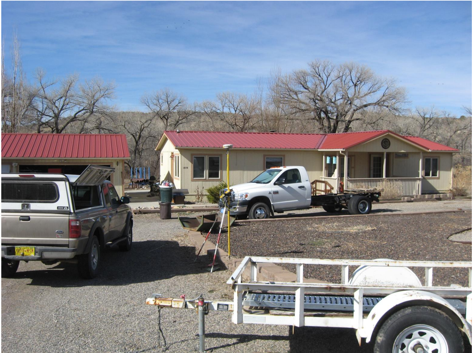
Front of structure looking West. 3/15/13
