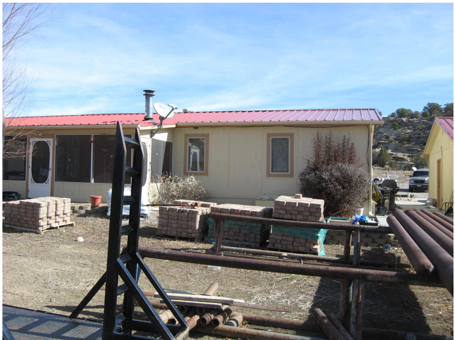
Back of structure looking East. 3/15/13
