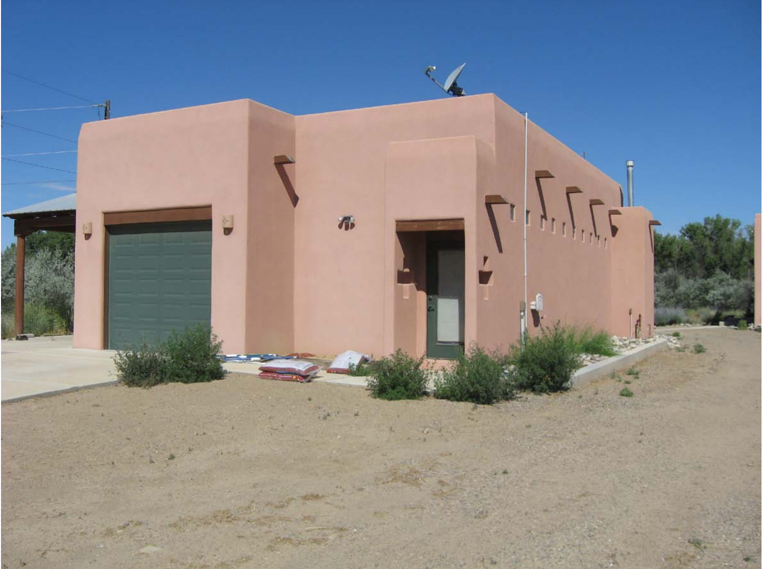
Back of stucture 2 looking West
