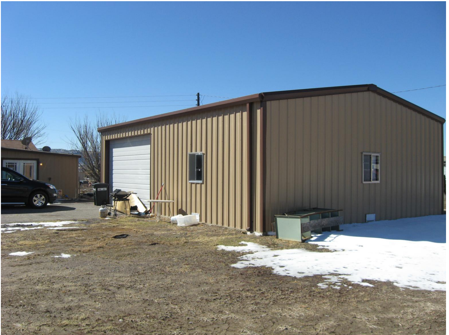
Front of structure looking Northwest 2/15/13
