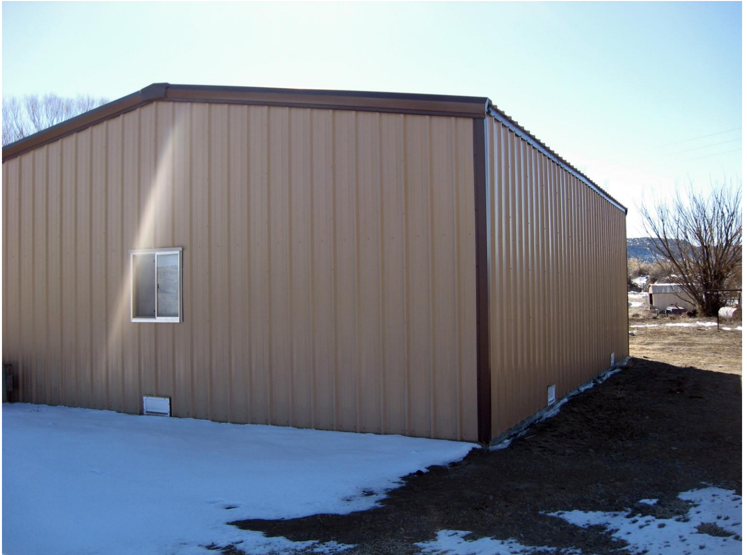
Back and side of structure looking West 2/15/13
