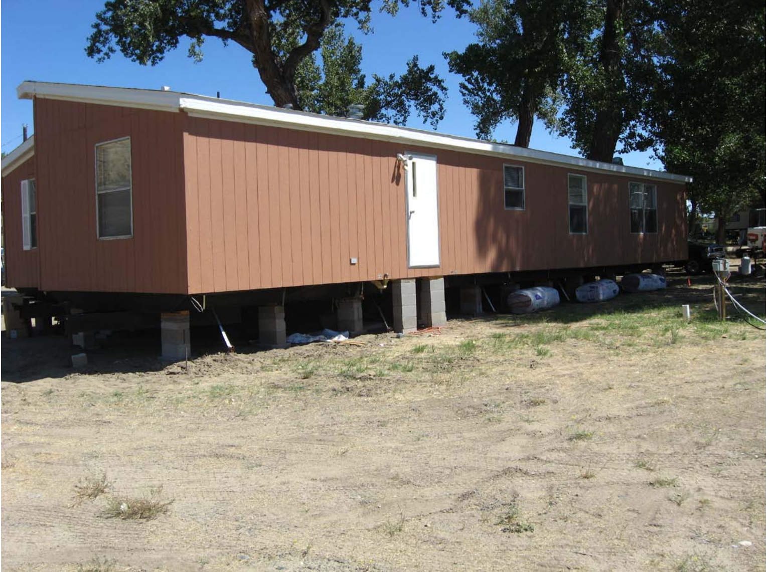
Back of structure looking West
