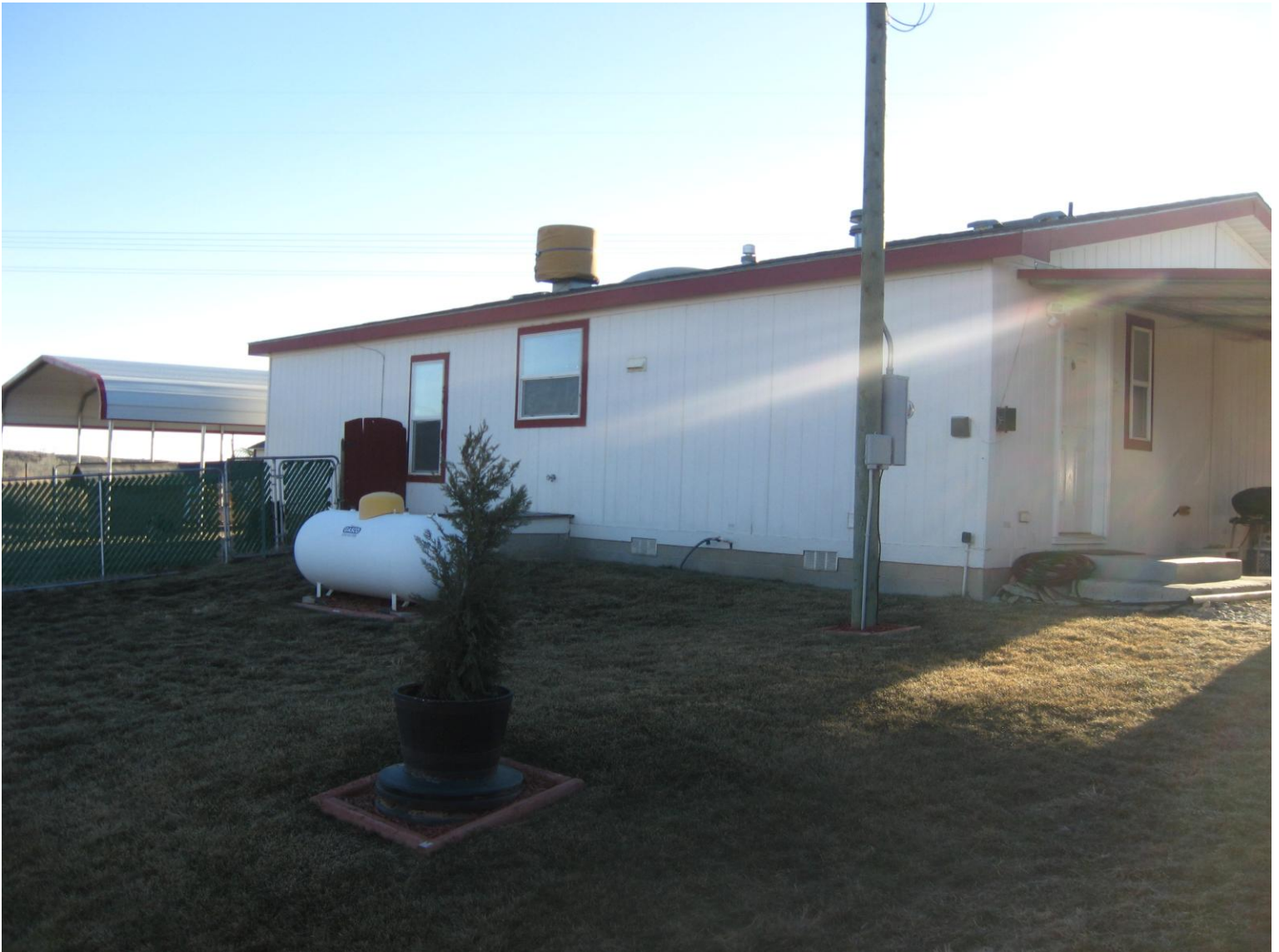
Back of structure, looking Southeast
