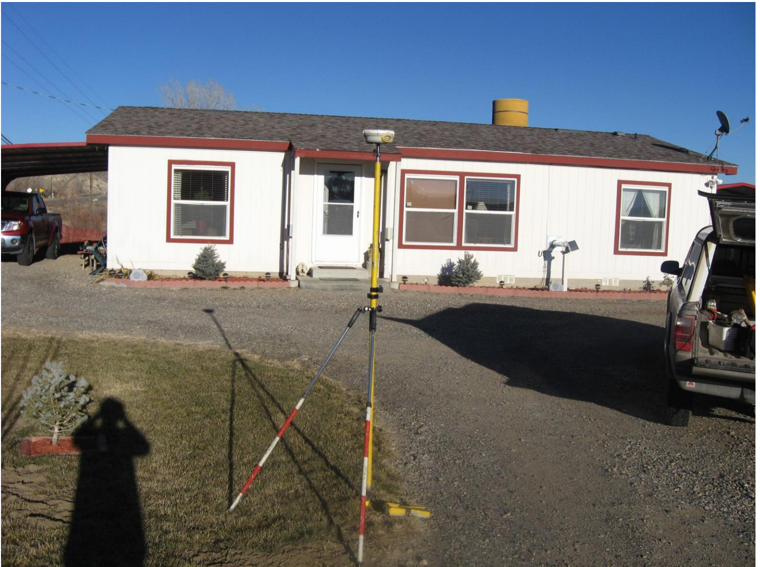
Front of structure, looking North
