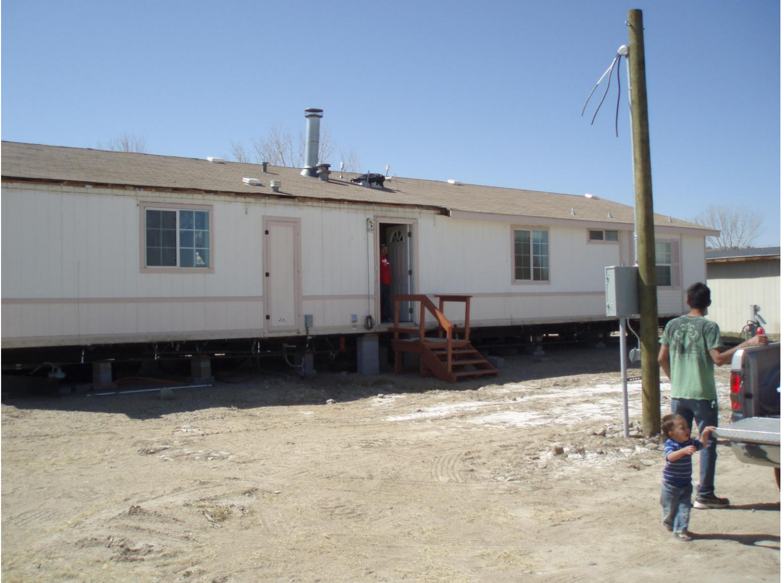
Back of structure, looking Southwest.
