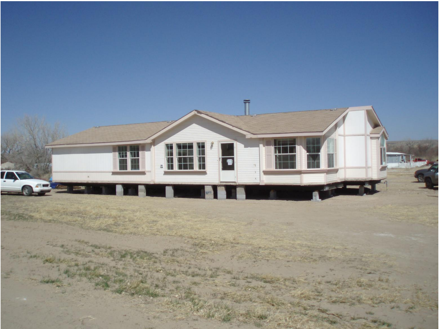
Front of structure, looking Northwest
