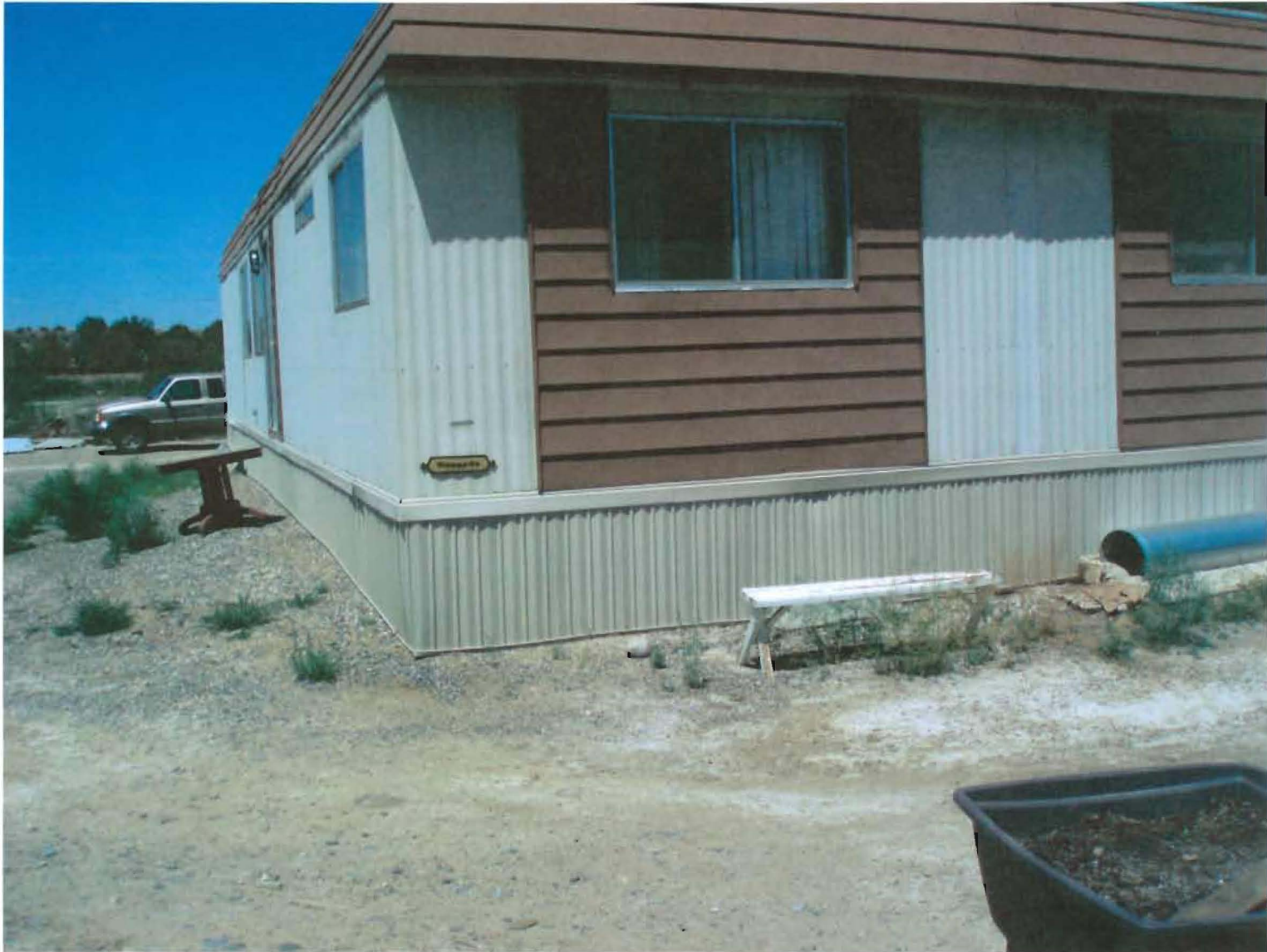
East end of structure looking West
