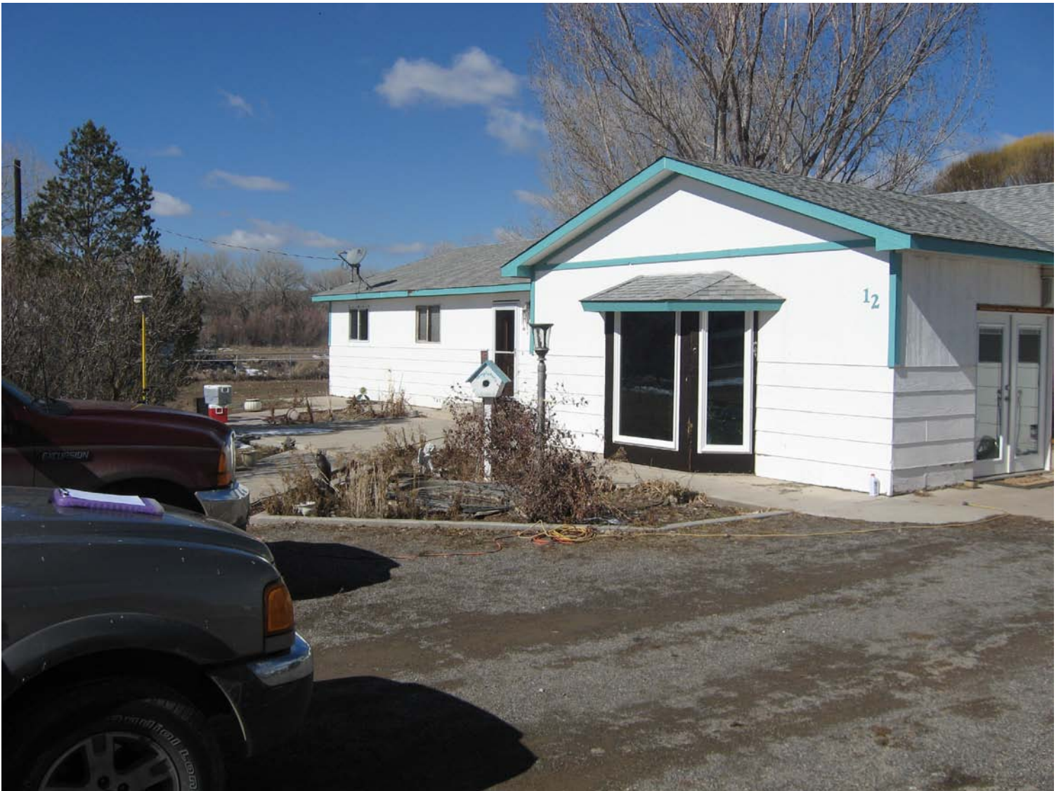
Front of House looking Northwest
