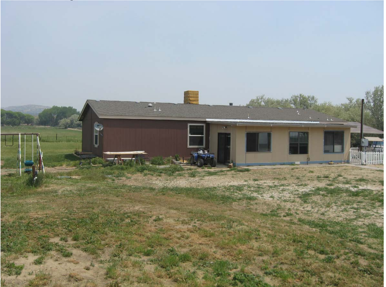
Rear of structure looking Northeast
