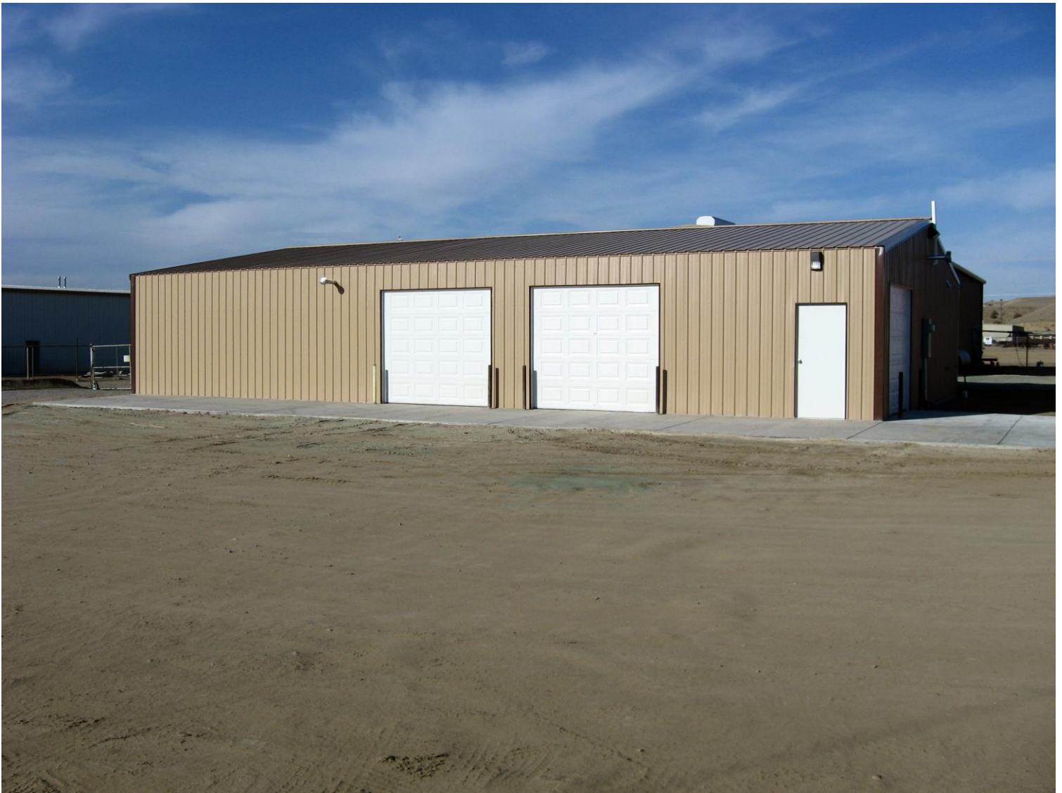
Front of building looking West
