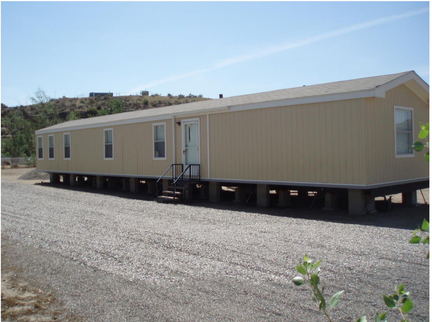
Front of structure, looking Southeast 7/12/2012
