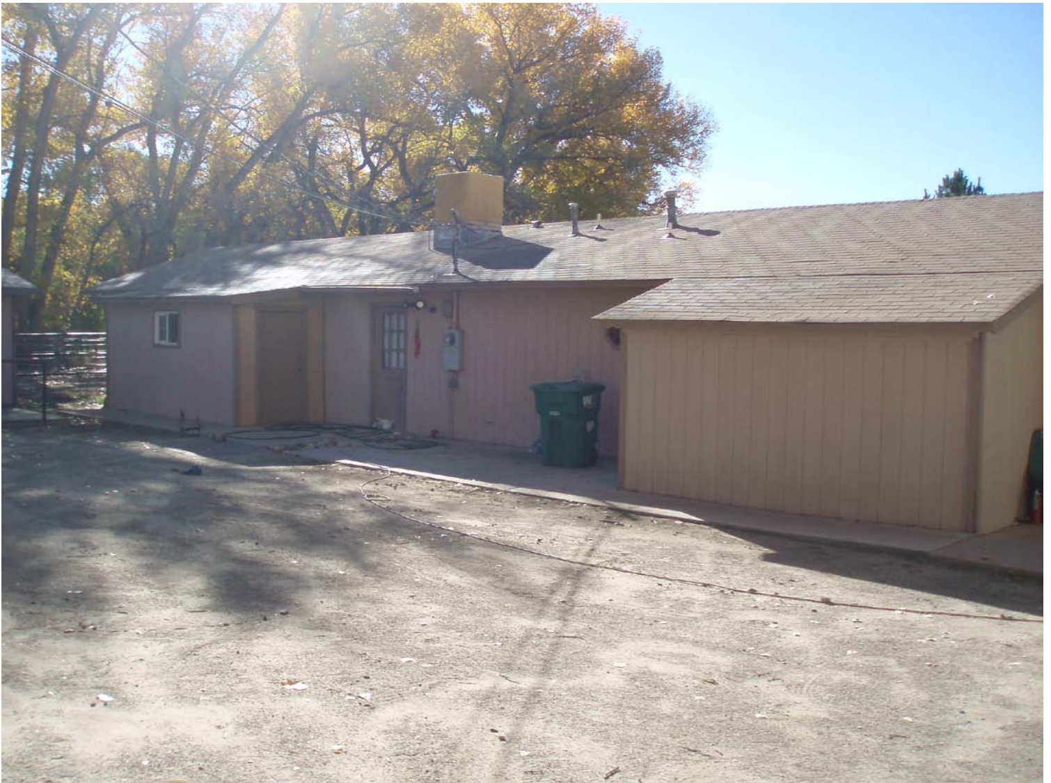
Back of House looking Southeast
