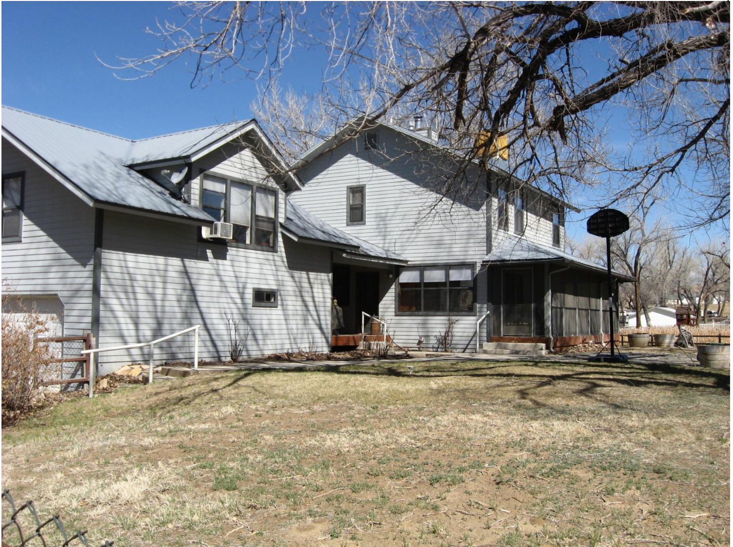
Back of structure looking North. 4/12/13
