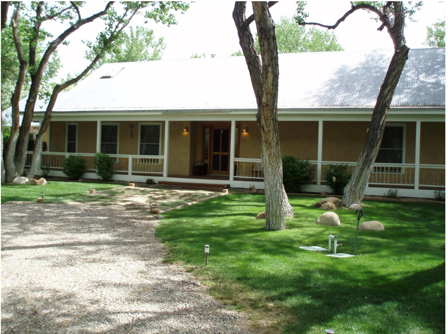
Front of structure, looking East
