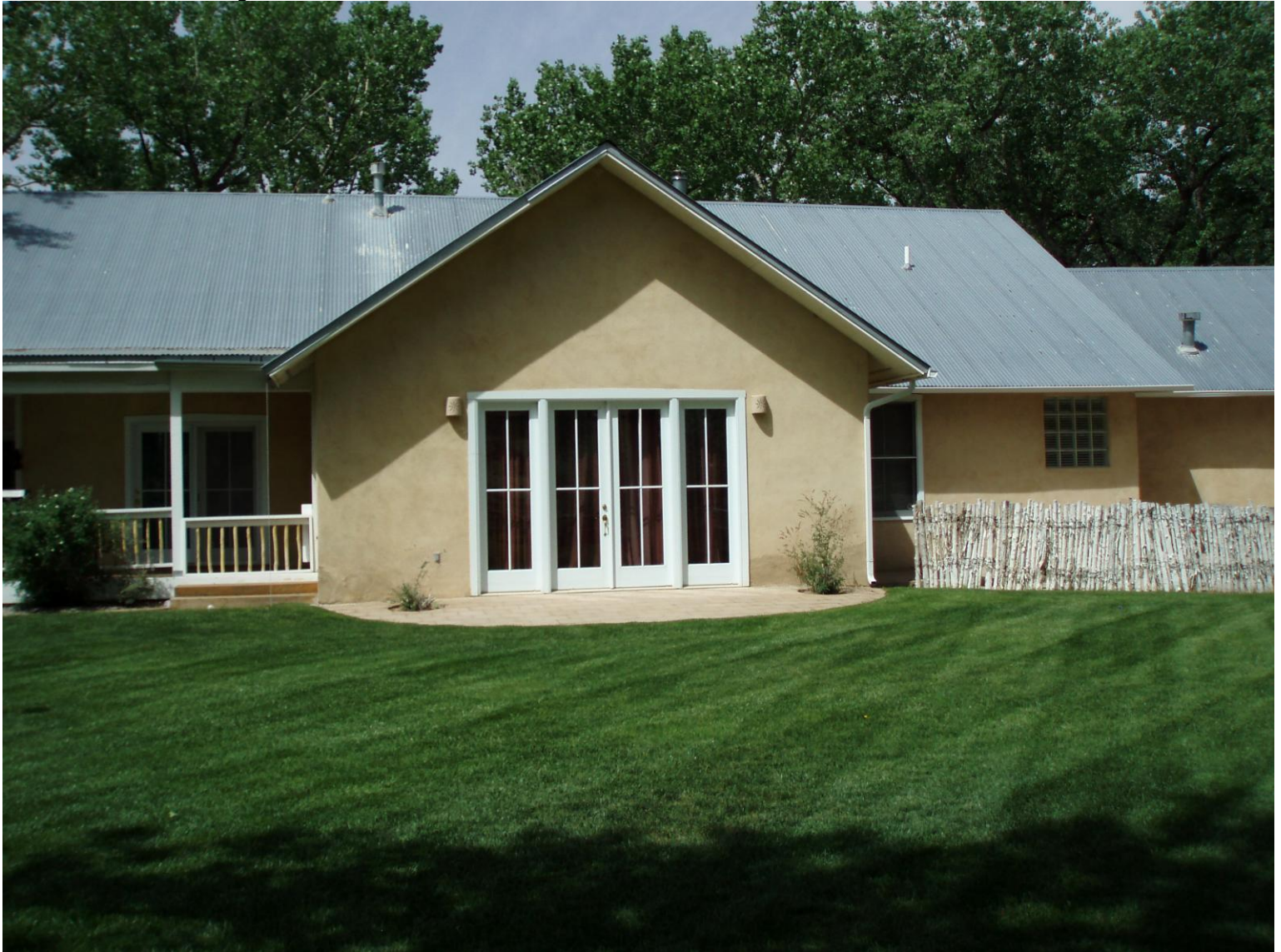
Back of structure, looking West
