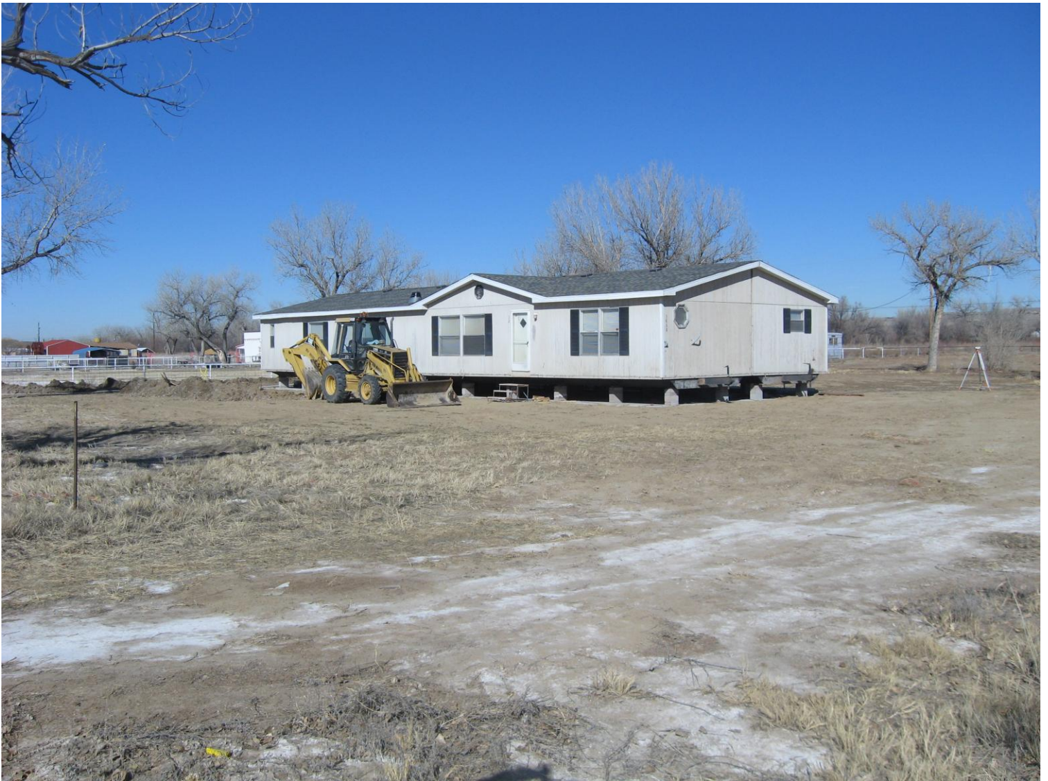
Front of structure, looking Northwest
