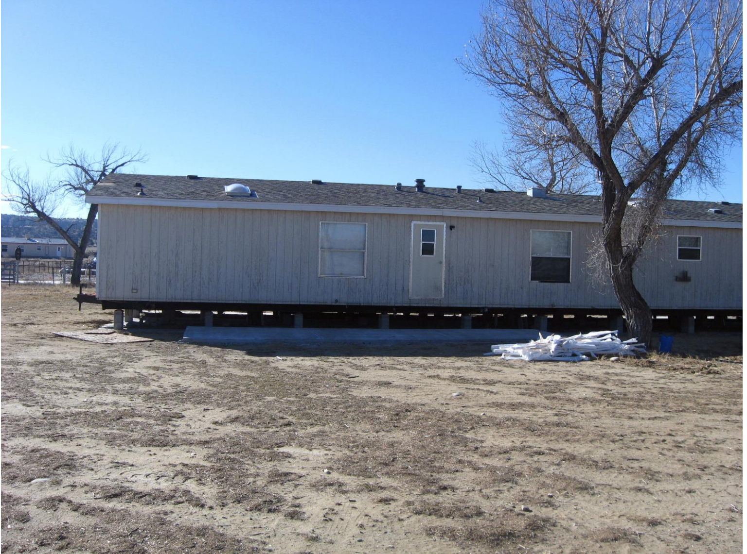
Back of structure, lookin South.
