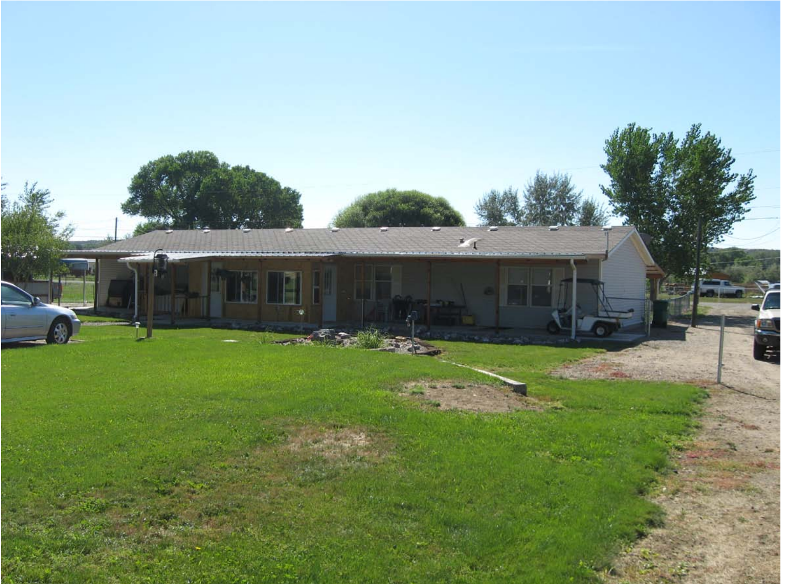
Back of structure lookin East
