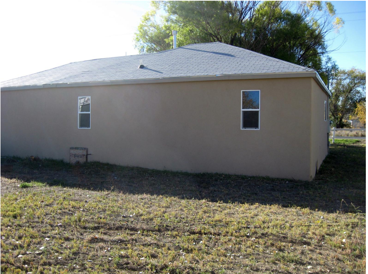
Back of structure looking South. 10/17/2012
