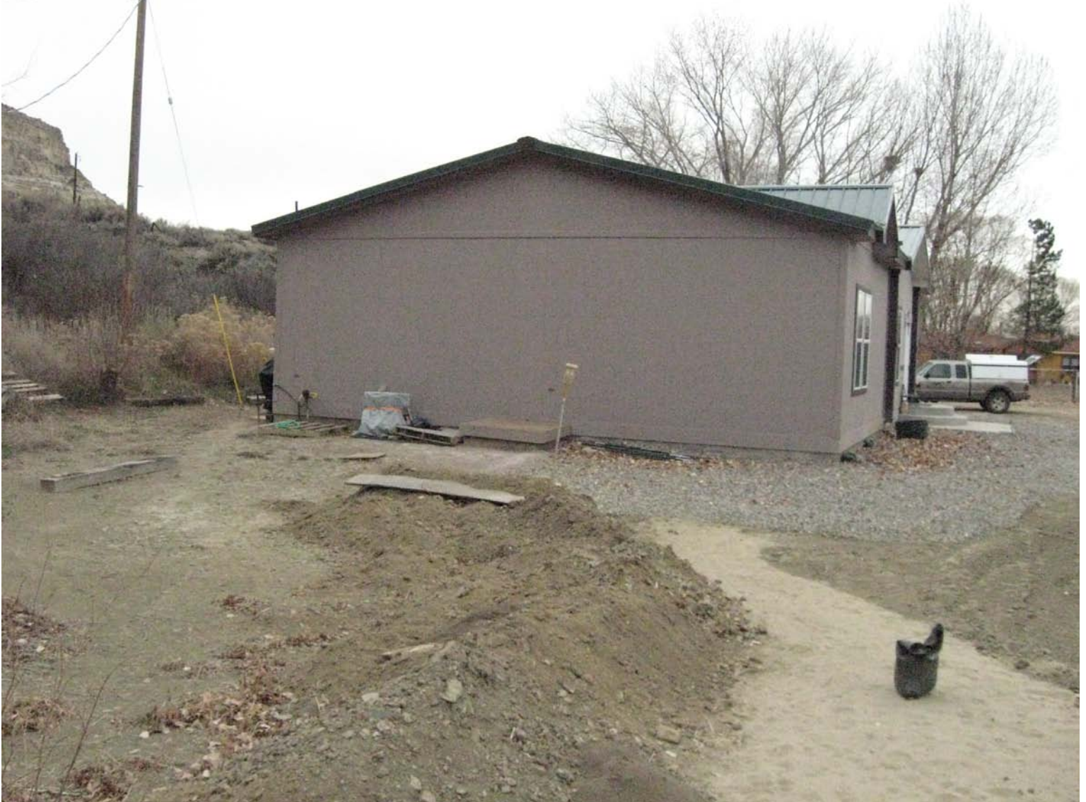
Side of building looking South
