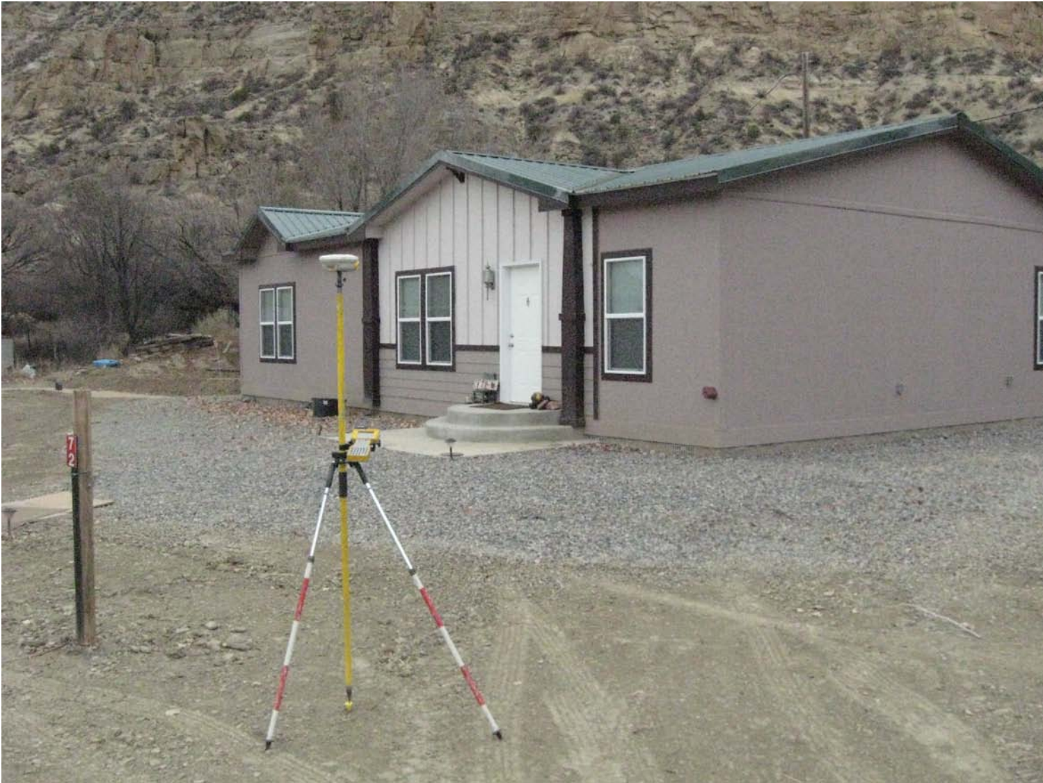
Front of building looking East
