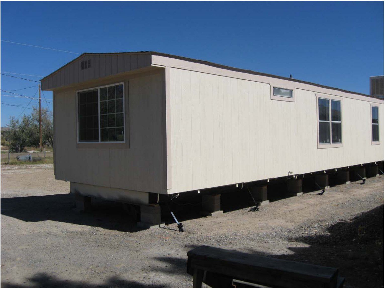
Back of structure Looking North
