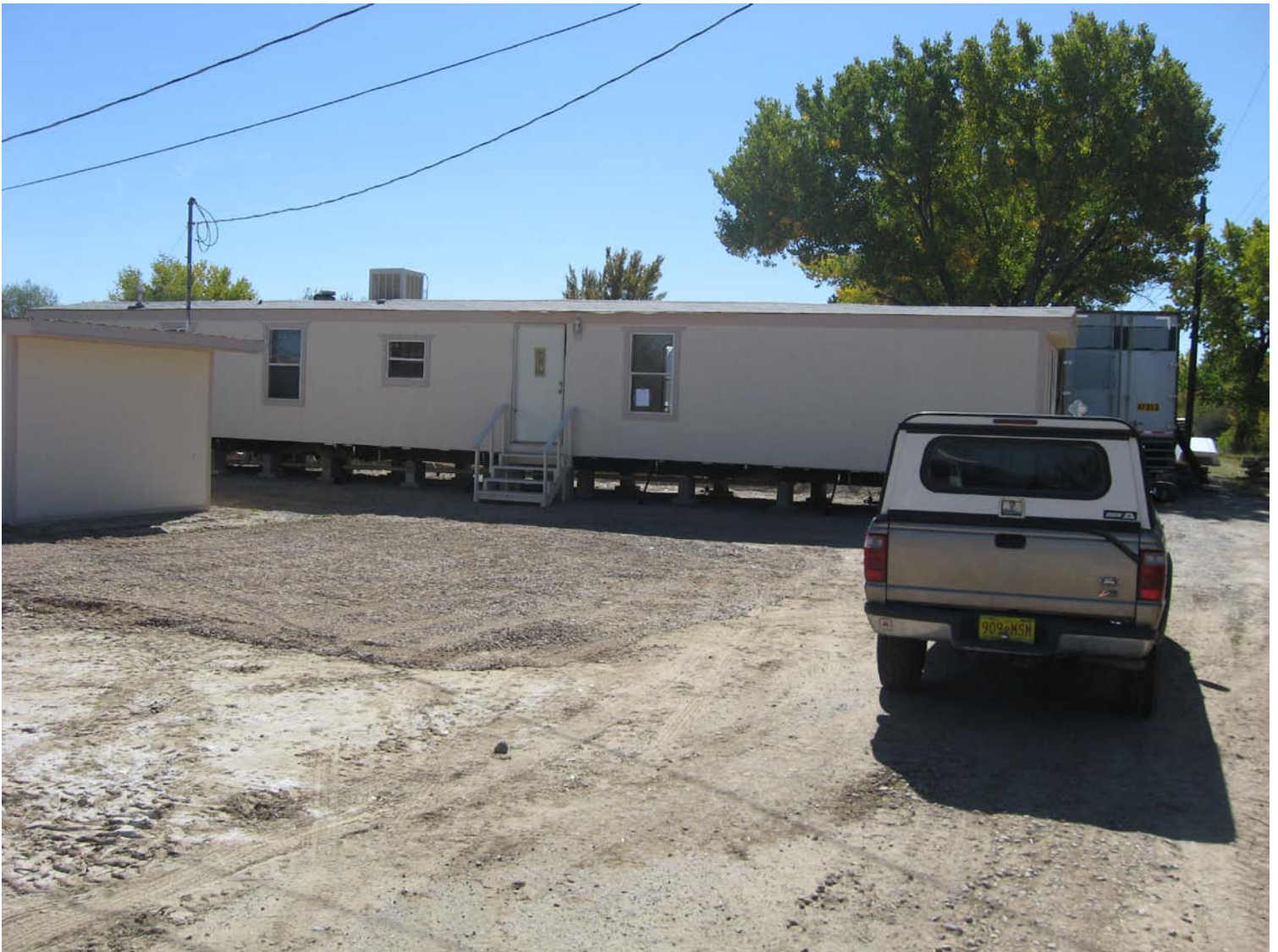
Front of structure looking South
