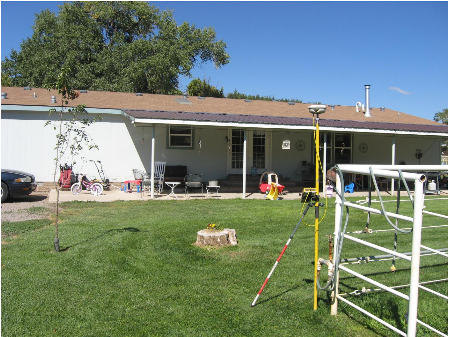
Front of structure looking West 9/13/2012
