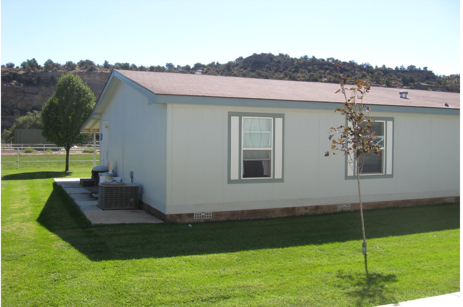
North and West side of structure 9/13/2012
