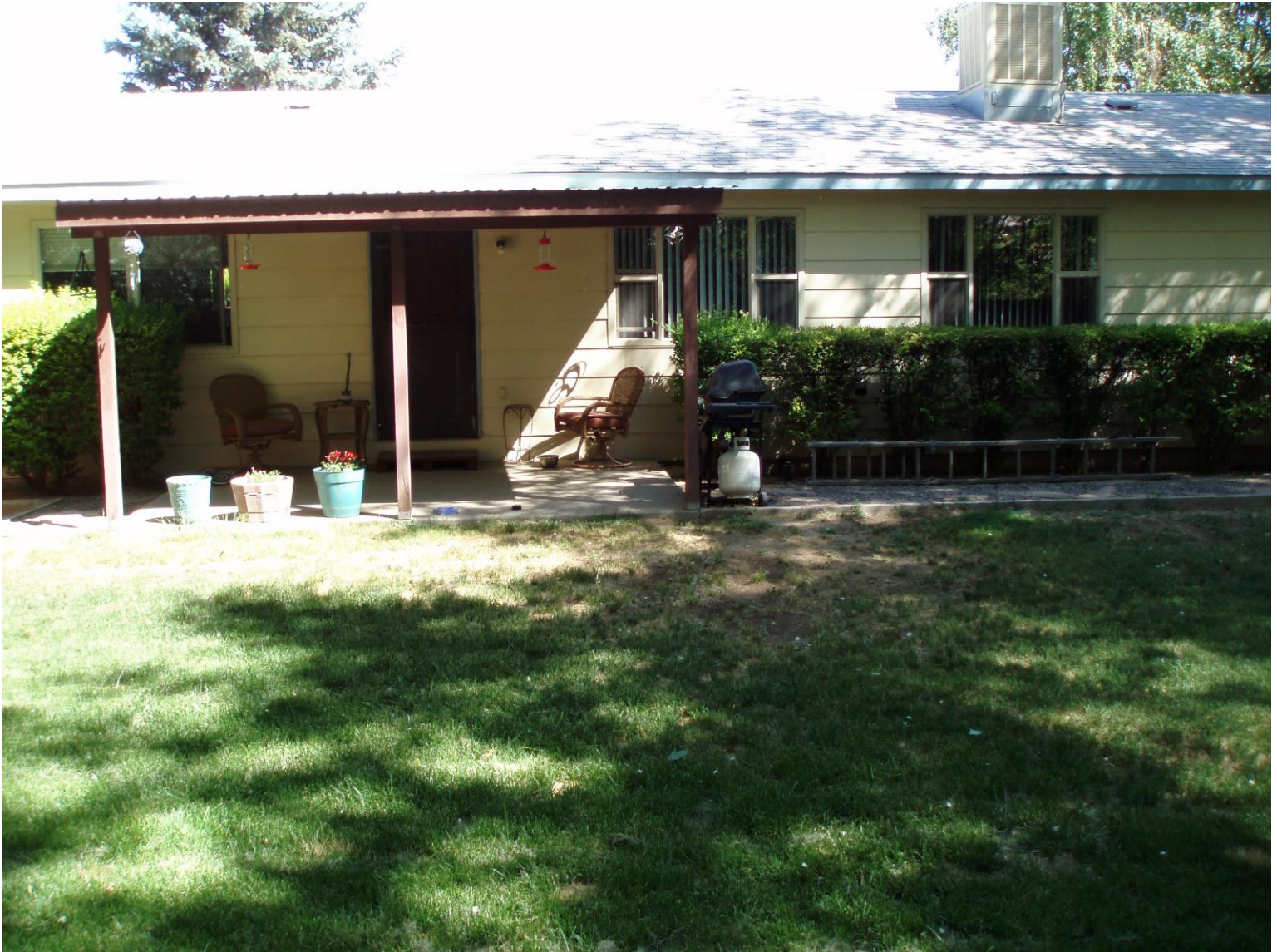
East side of structure
