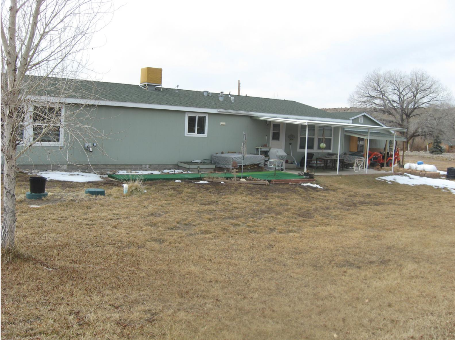
Back of structure looking Southwest
