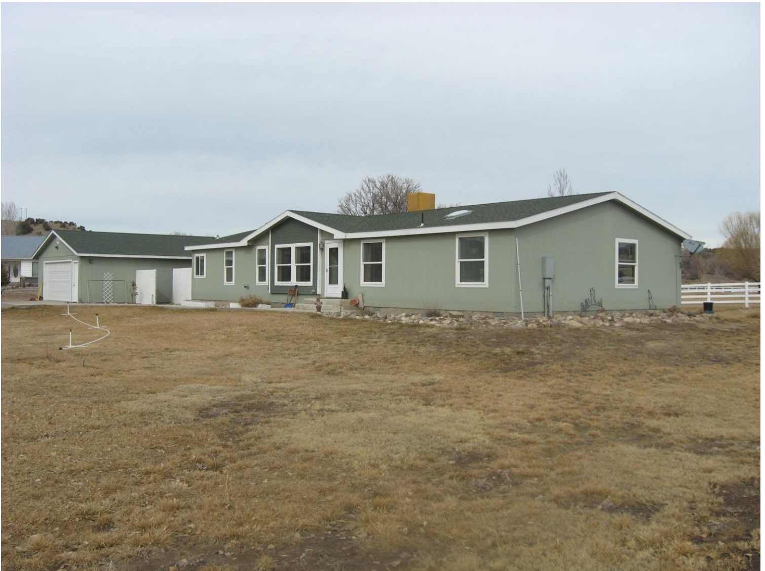
Front of structure looking Northwest
