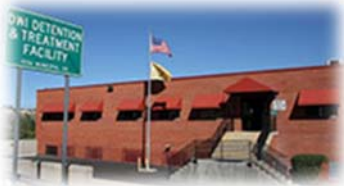
DWI Detention & Treatment Facility Farmington, NM
