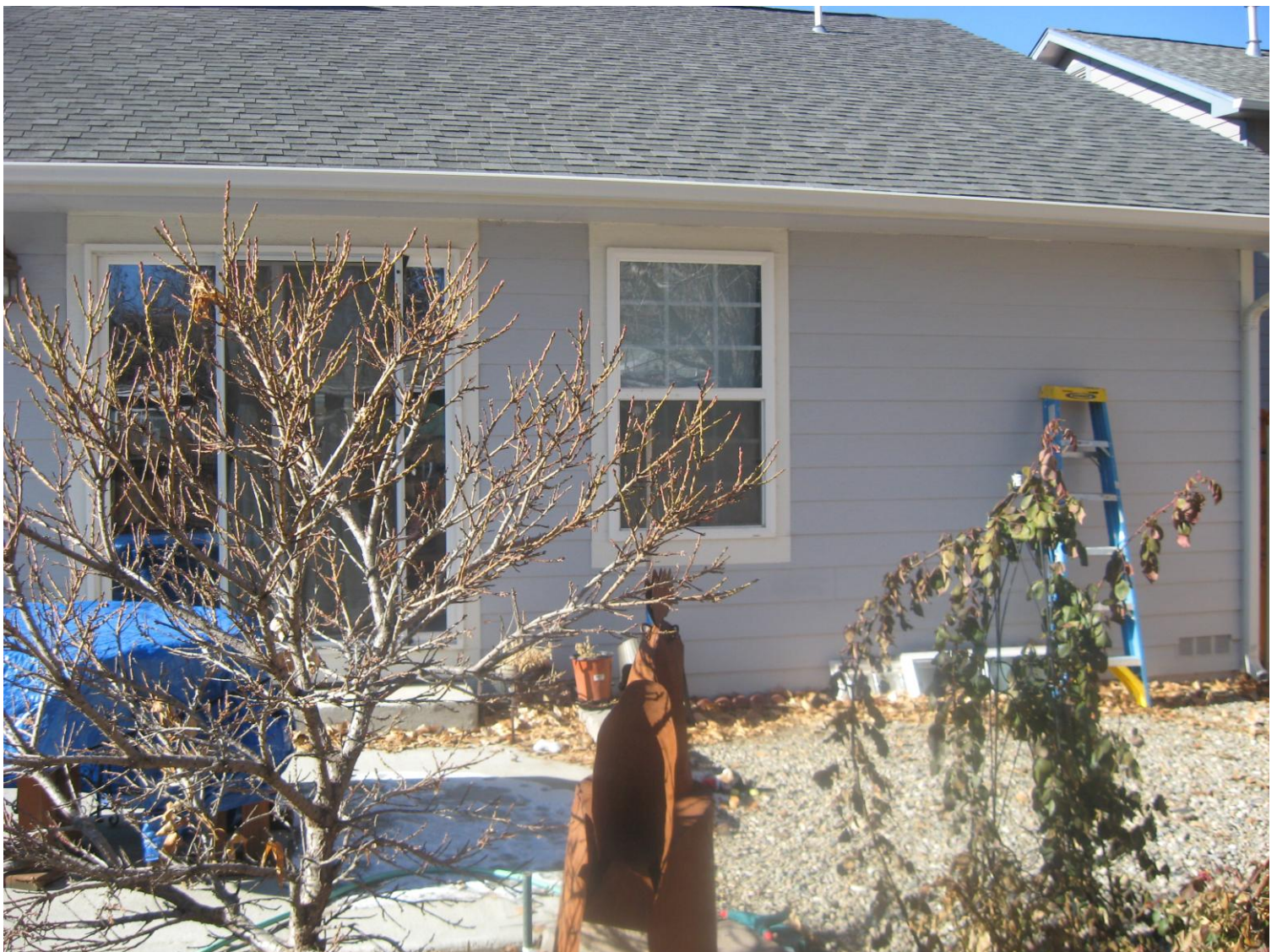
Back of house looking West
