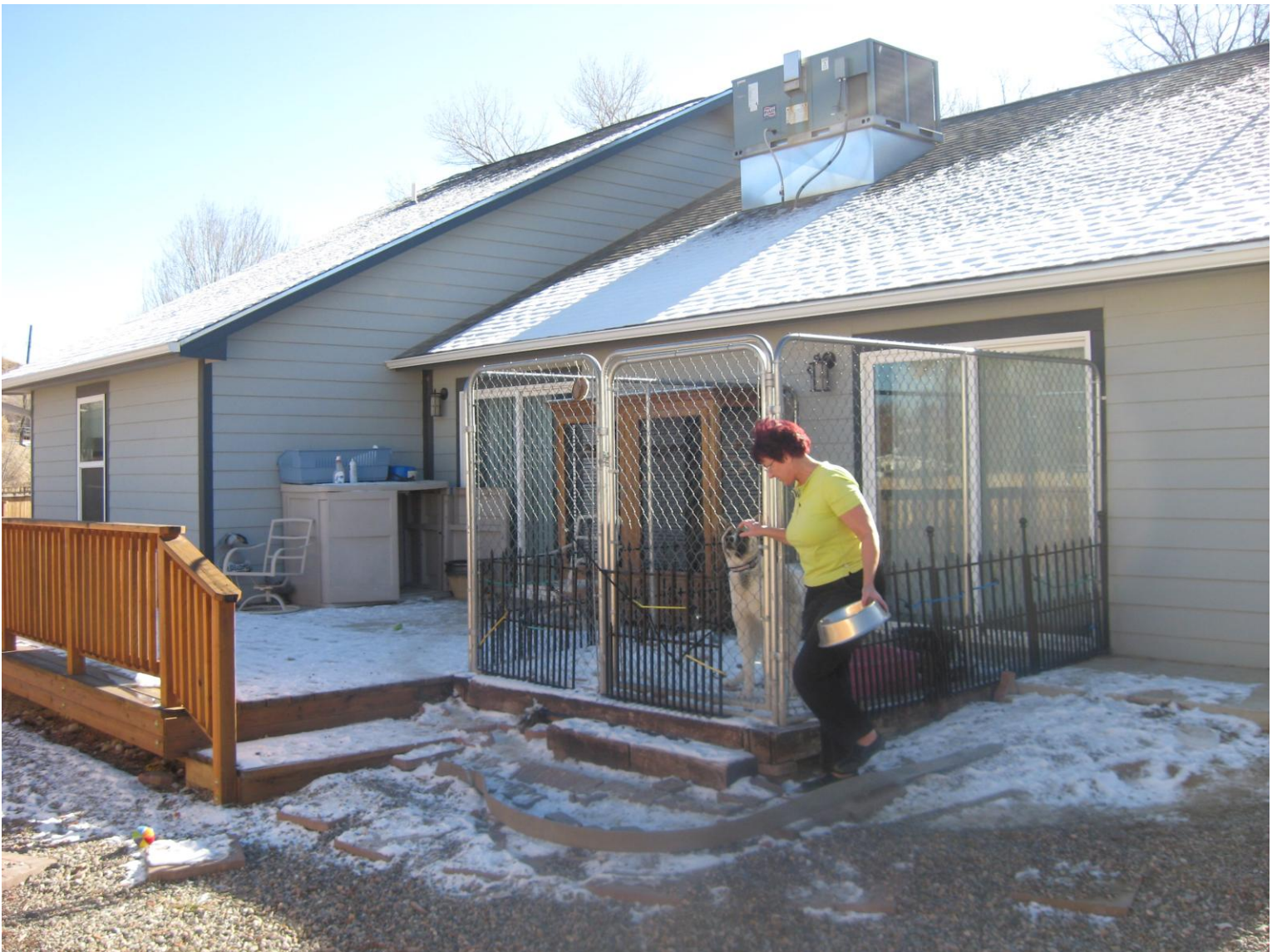
Back of house, looking Southeast
