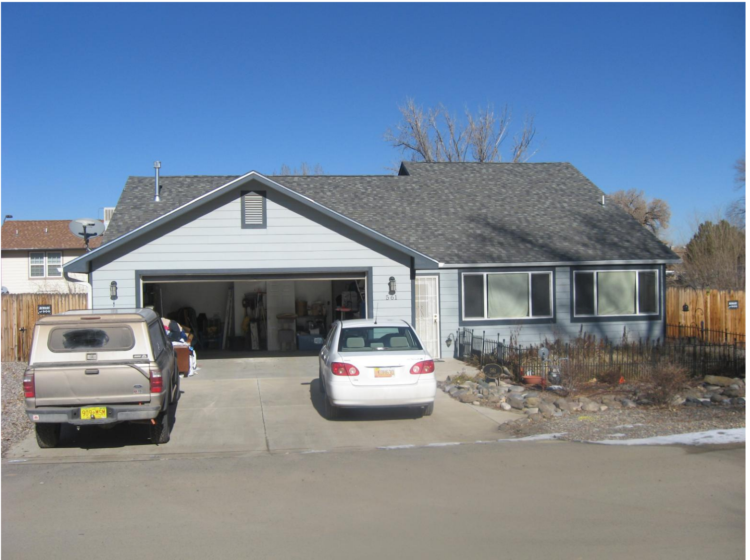
Front of house looking North
