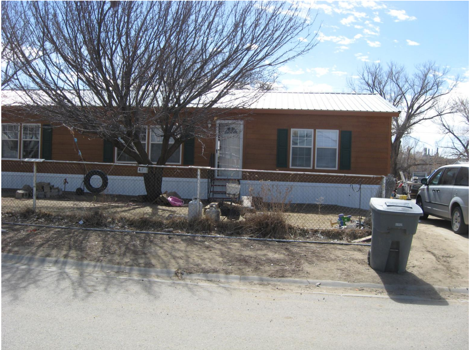
Front of structure looking South. 3/6/13
