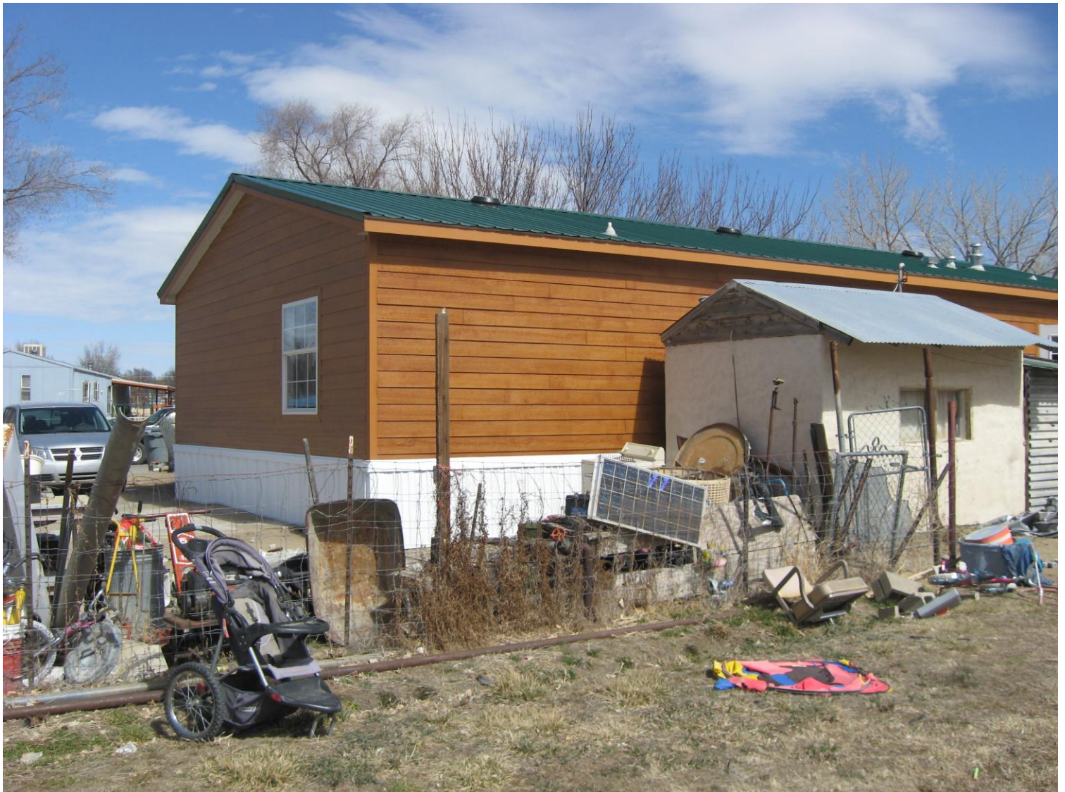
Back of structure looking NE. 3/6/13
