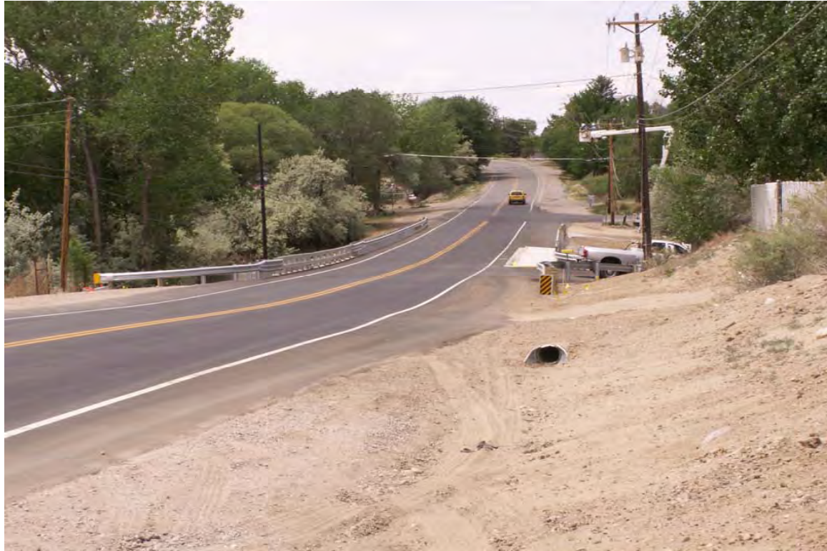
New Bridge - Kirtland, NM
