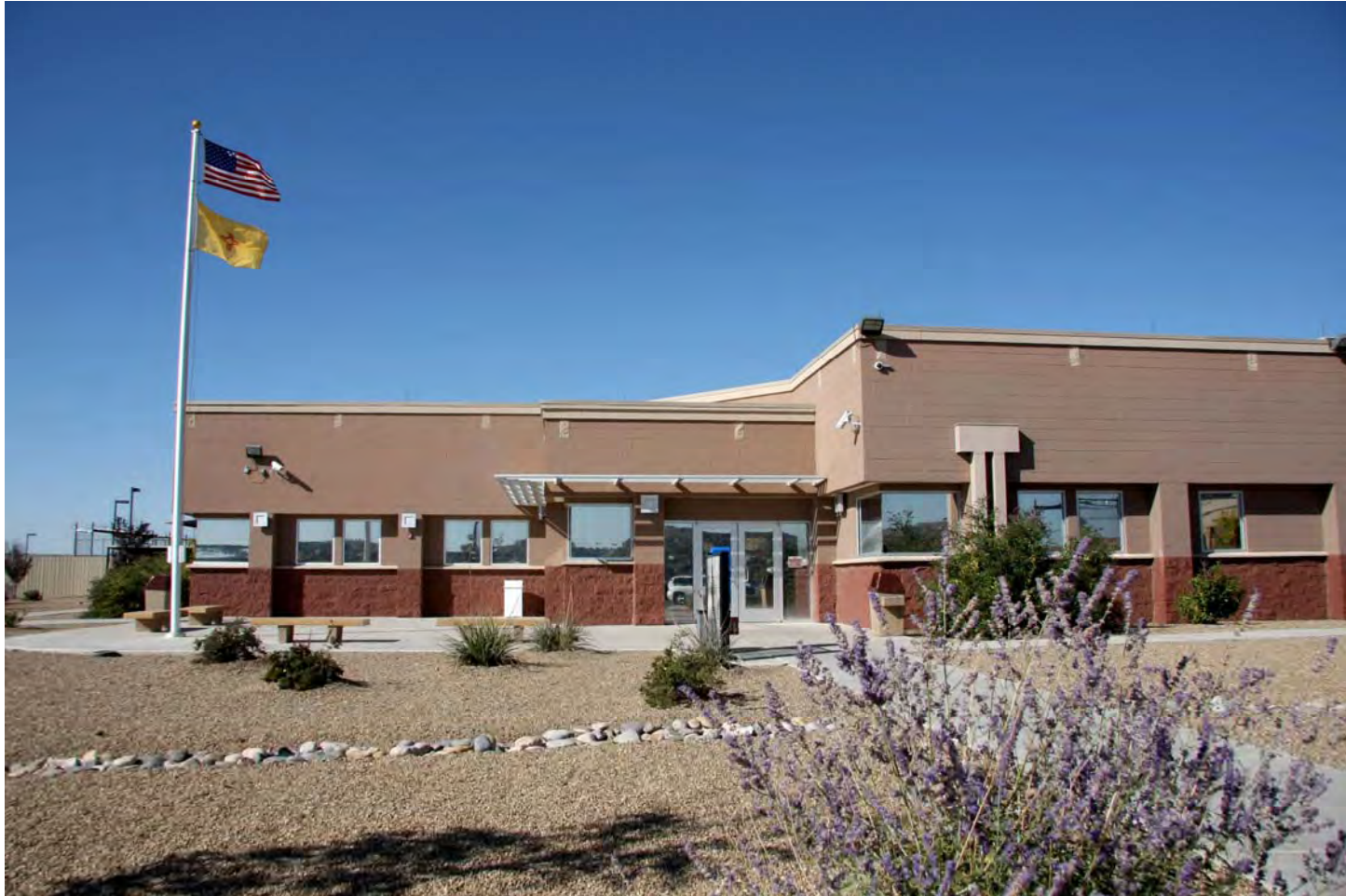
San Juan County Detention Center
