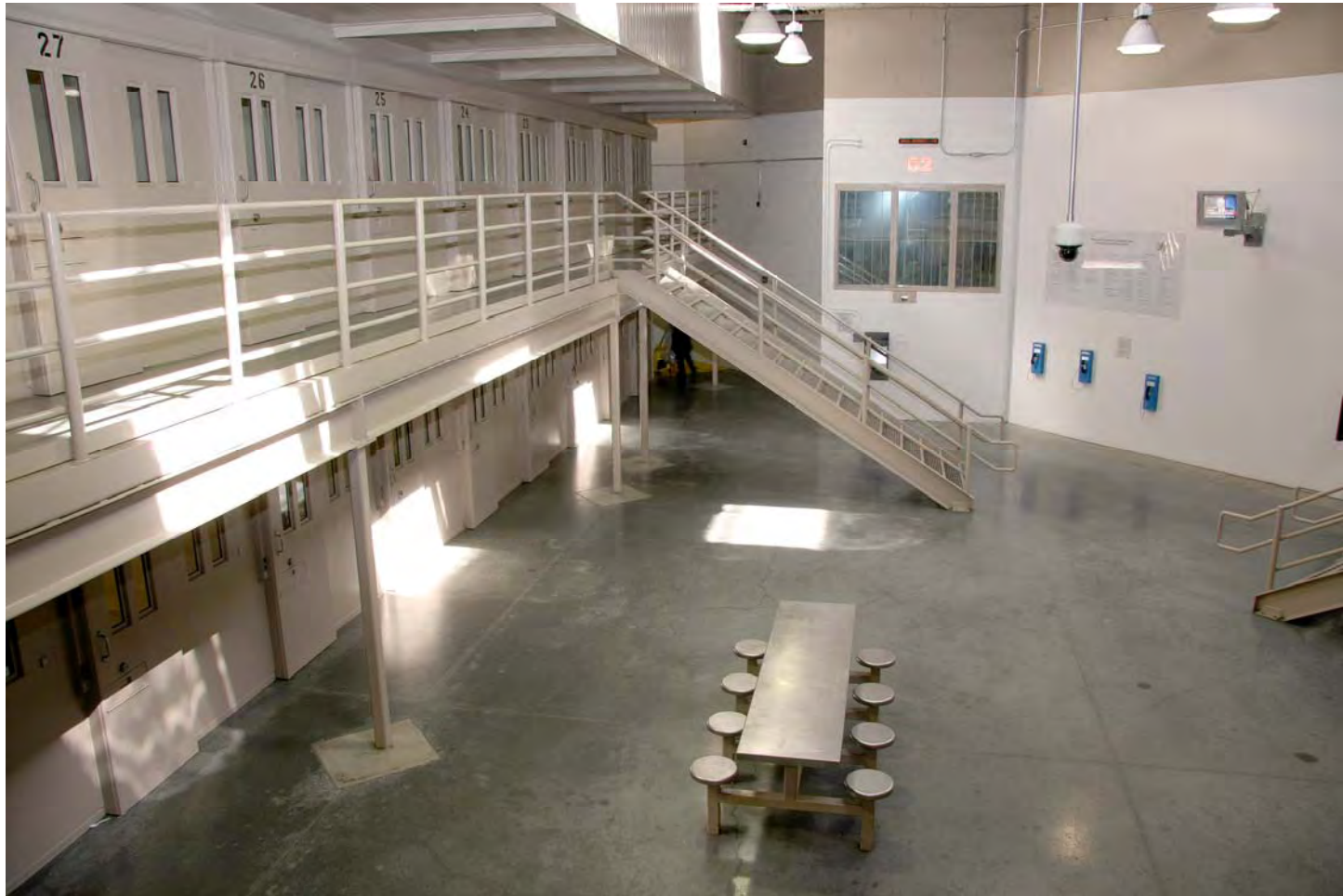
San Juan County Detention Center
