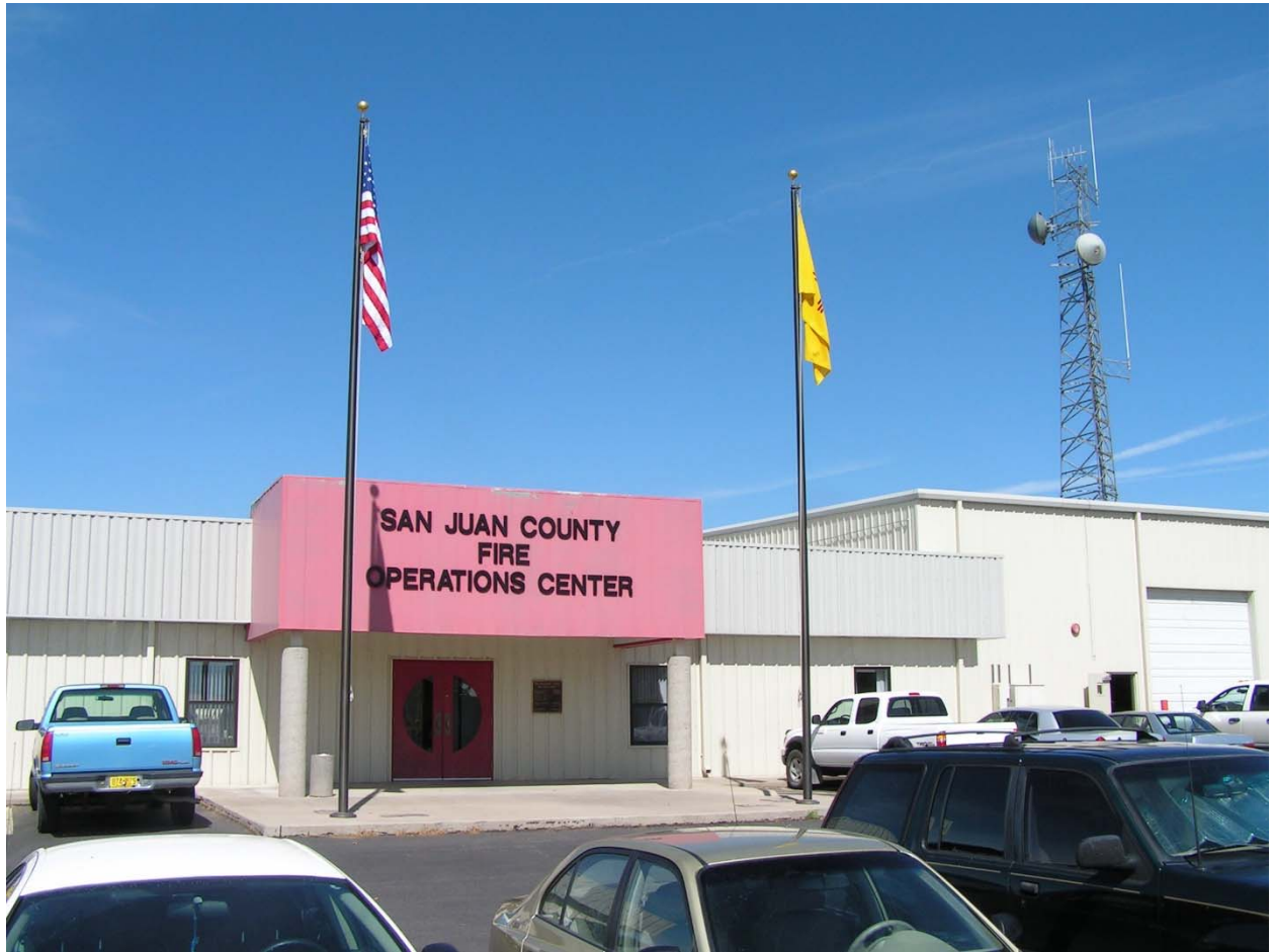
San Juan County Fire Operations Center
