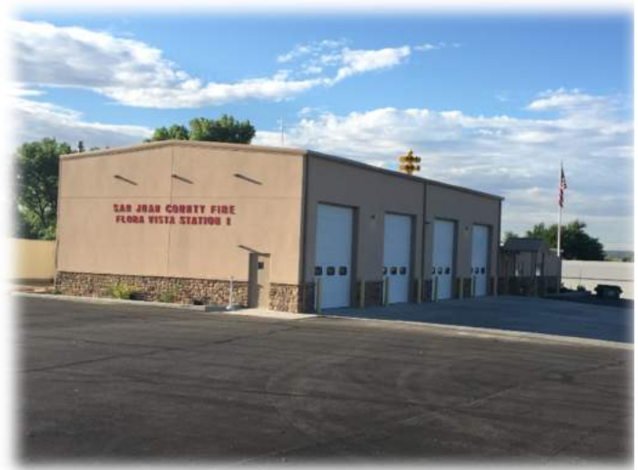
Flora Vista County Fire Station, Flora Vista, NM
