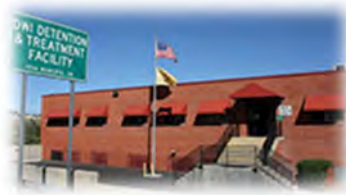
DWI Detention & Treatment Facility Farmington, NM
