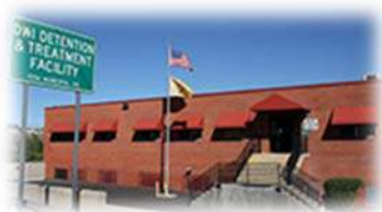
DWI Detention & Treatment Facility Farmington, NM
