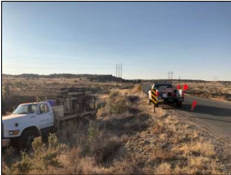
Drill Rig at Boring B-15 View towards the Southeast
