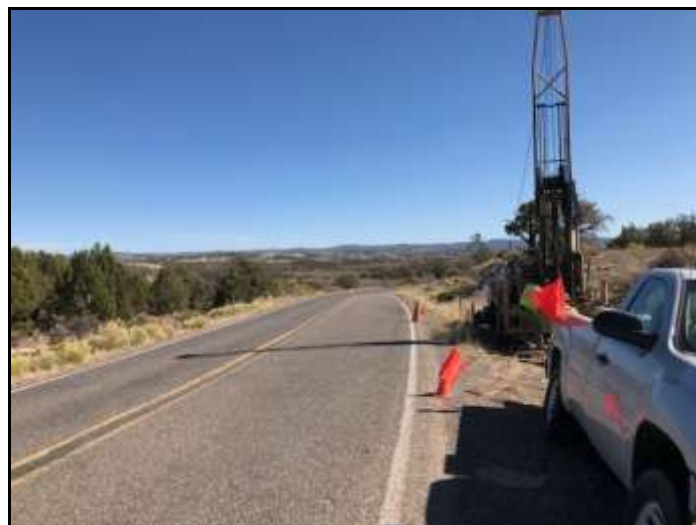
Drill Rig at Boring B-7 View Towards the Southeast
