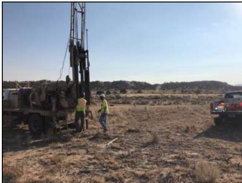
Drill Rig at Boring B-19 View towards the East
