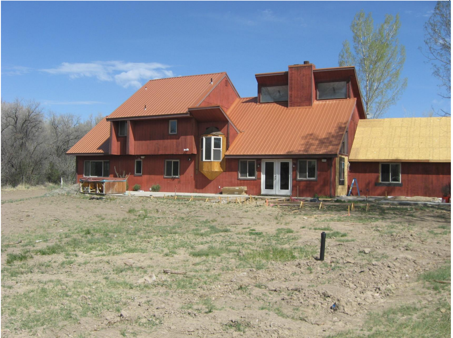
Front of structure looking North, 5/1/13
