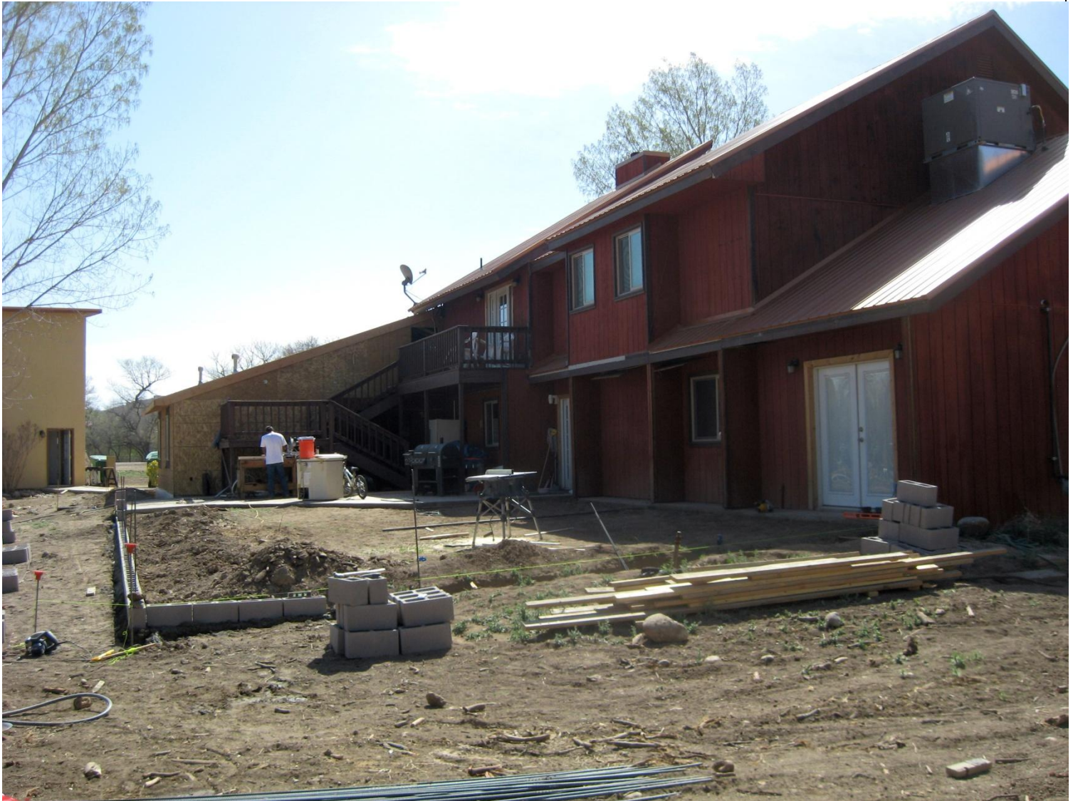
Back of structure looking Southeast, 5/1/13
