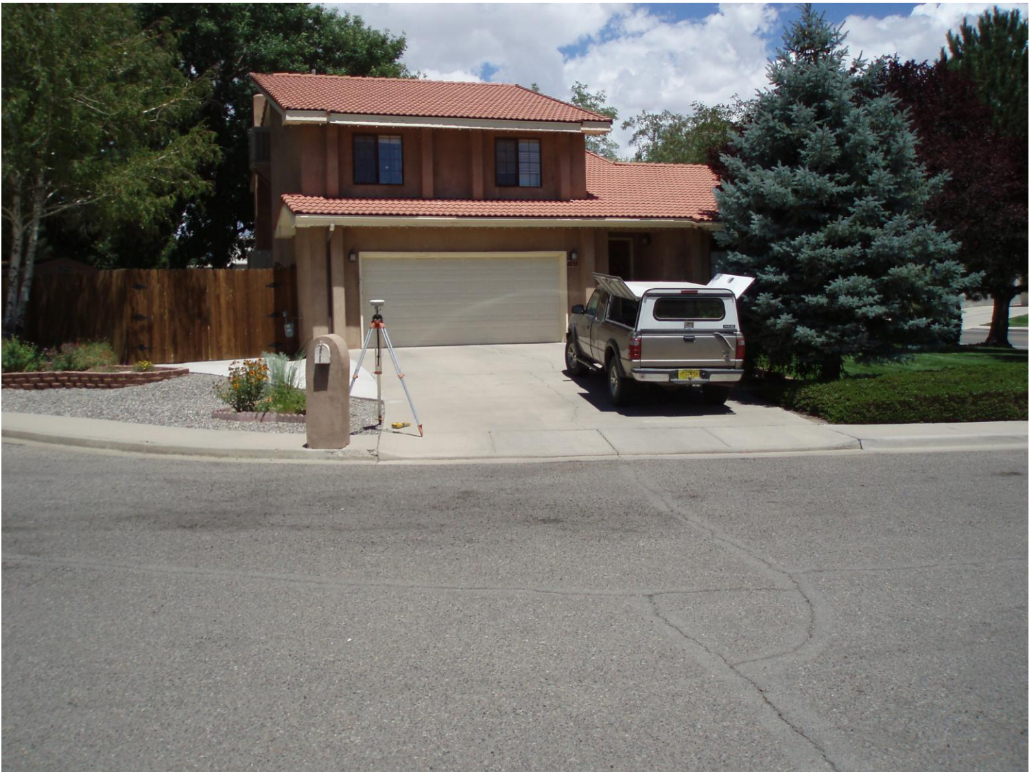
Front of structure looking North. 7/25/2012
