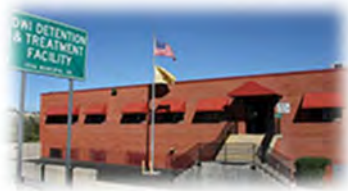
DWI Detention & Treatment Facility Farmington, NM
