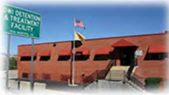
DWI Detention & Treatment Facility Farmington, NM
