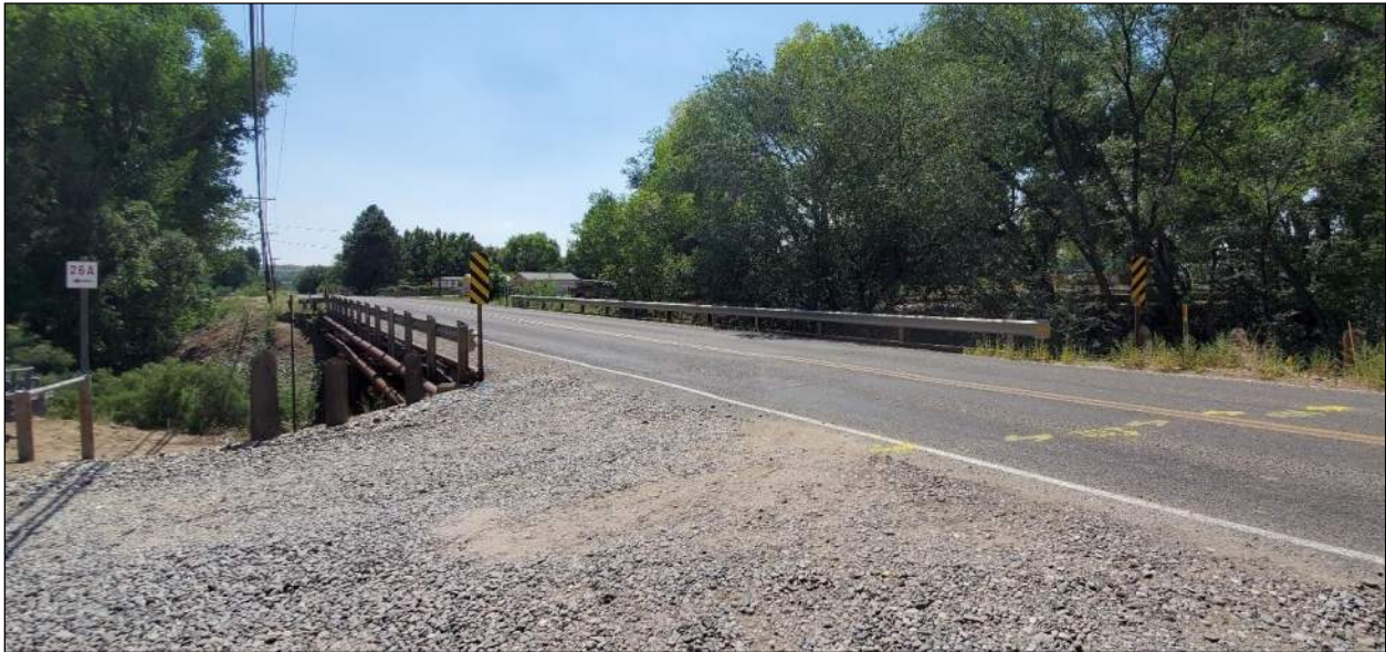
Photograph 3: BR 8111 View to the South
