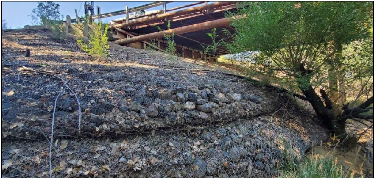
Photograph 4: BR 8111 Underside and Embankment Stabilization View to the Southwest
