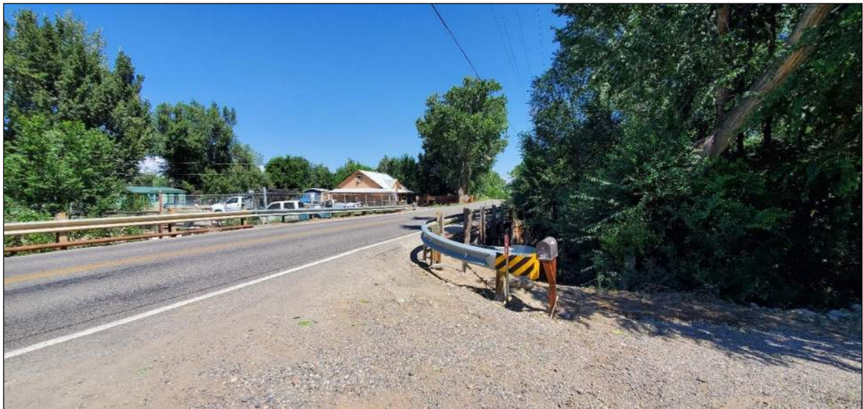
Photograph 1: BR 3121 View to the North
